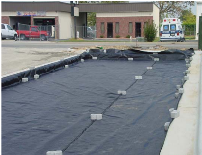
Figure VIII: Permeable pavement with geotextile to prevent contamination of the base layer at bottom and sides
