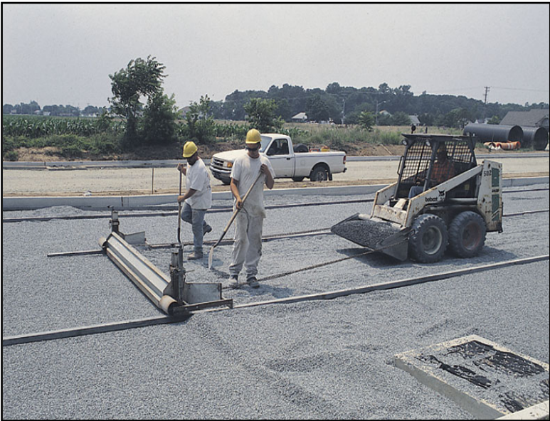
Figure X: Mechanical screeding of the No. 8 bedding layer (Source: ICPI, 2000)
