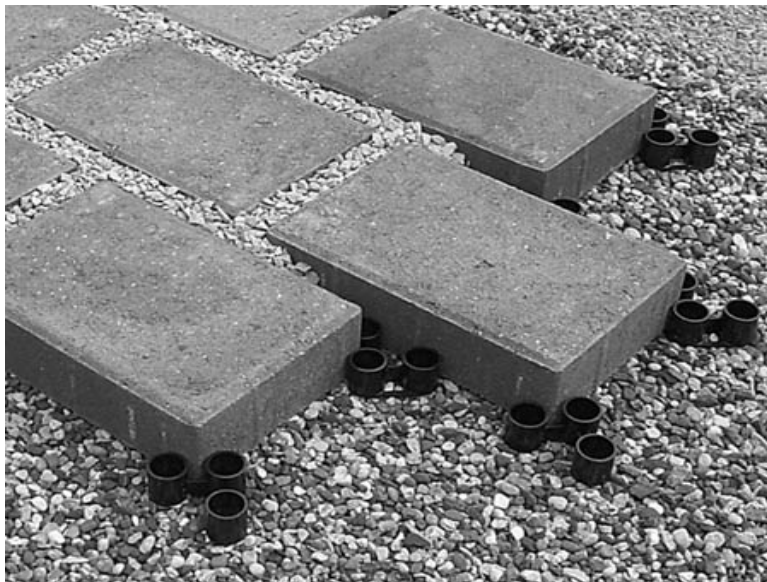
Figure VI: Plastic spacers are used to create enlarged permeable joints (Source: ICPI, 2000)
