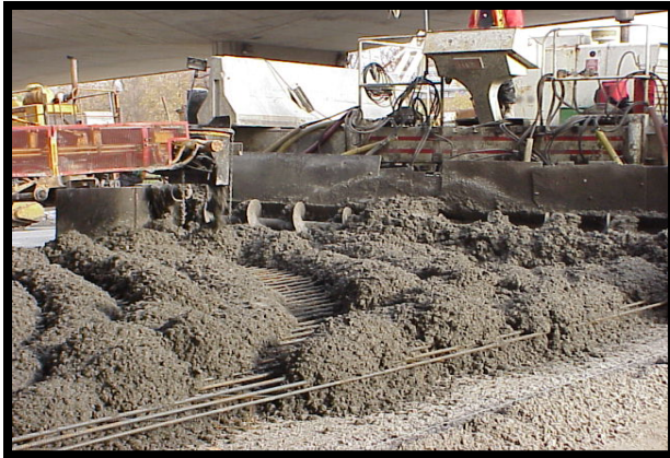
Figure 4 – Construction of CRCP
