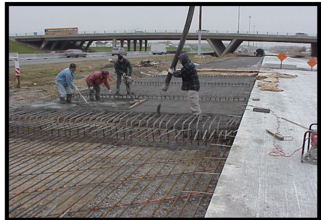
Figure 2 – Placement of the transversal and longitudinal reinforcement
