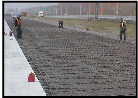
Figure 2 – Placement of the transversal and longitudinal reinforcement
