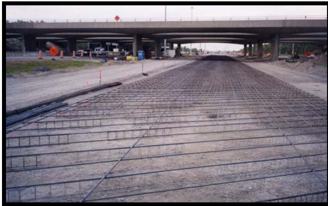
Figure 2 – Placement of the transversal and longitudinal reinforcement
