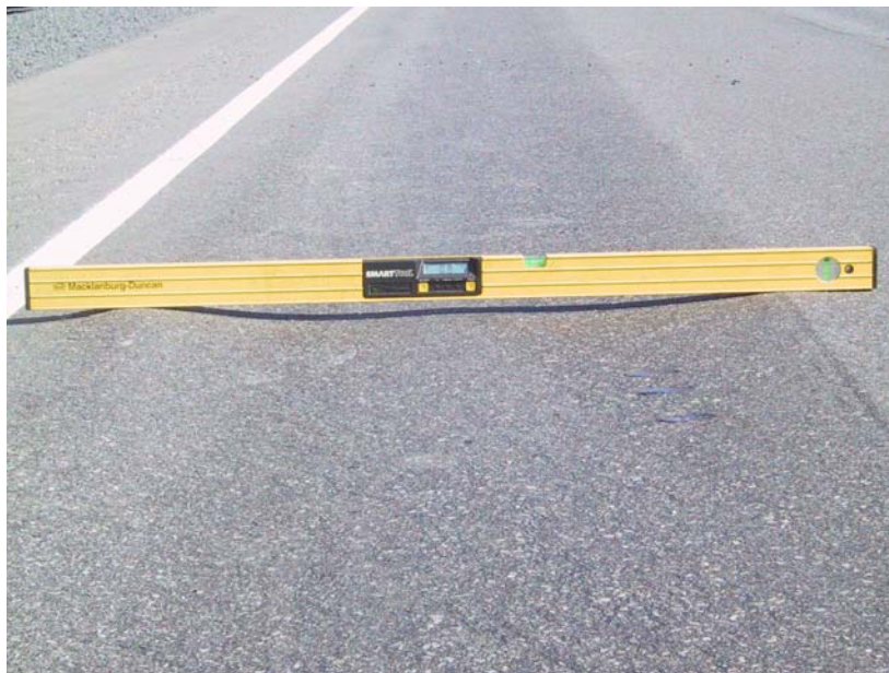
PHOTOGRAPH 1 Asphalt pavement rutting due to plastic movement of the asphalt mix under heavy loads.
