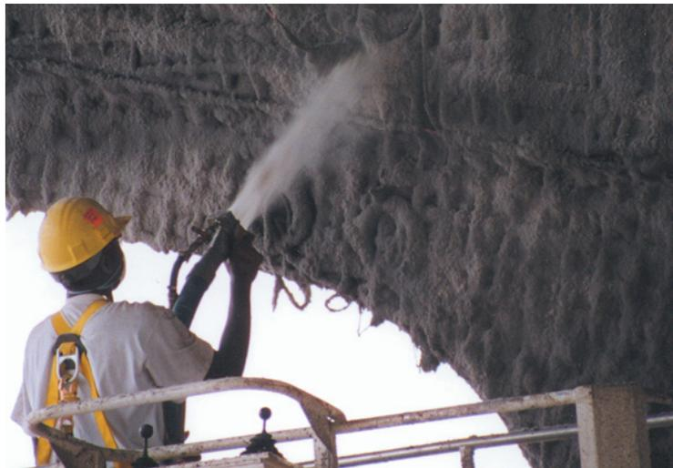
Figure 8: Cellulose Fiber Mixture Sprayed onto Surface of Concrete
