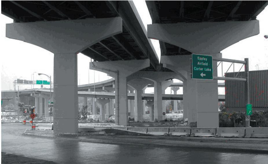
Figure 9: Completed Repair And Rehabilitation of I-480 Viaduct Substructure
