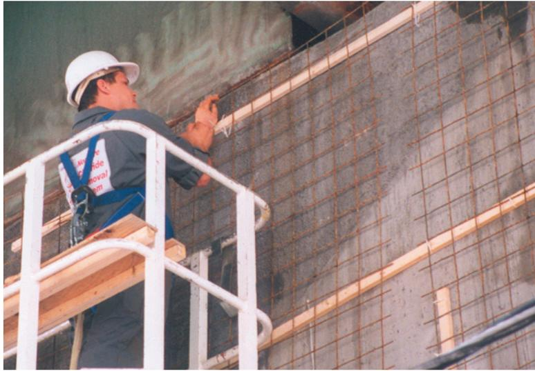
Figure 7: Electrode Mesh Installed on Surface of Piers
