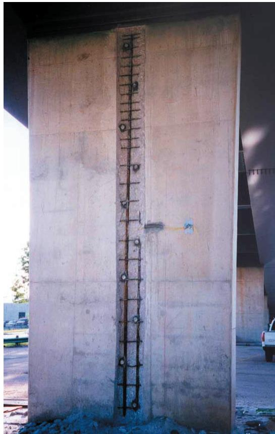
Figure 6: Embedded Galvanic Anodes Installed in I-480 Pier
