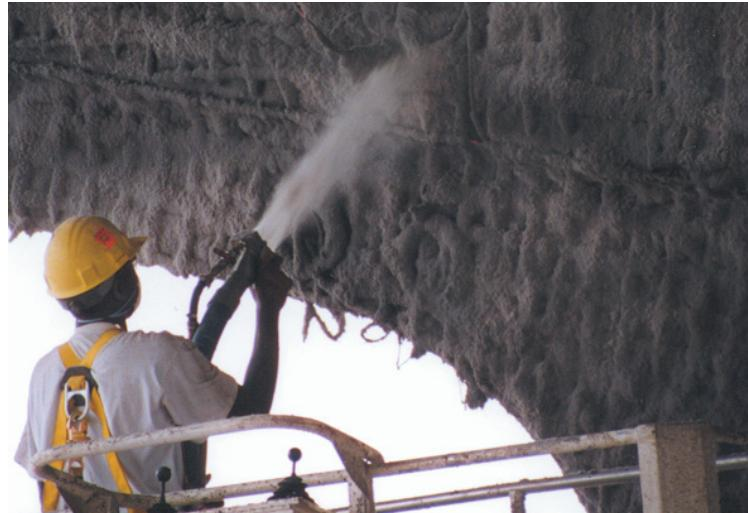
Figure 8: Cellulose Fiber Mixture Sprayed onto Surface of Concrete
