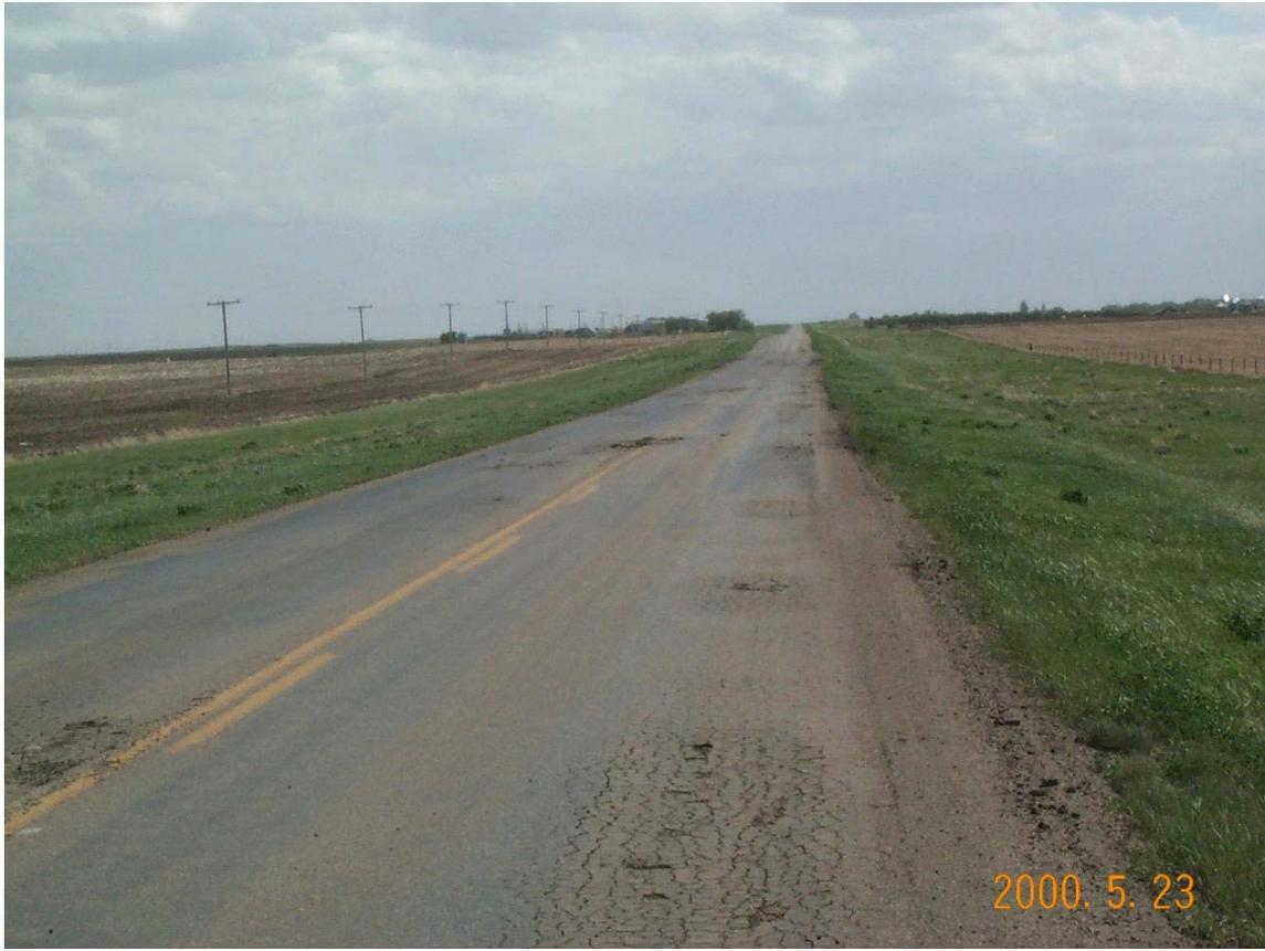
**Figure 4 – Pre-construction Road Condition on Highway 19**
