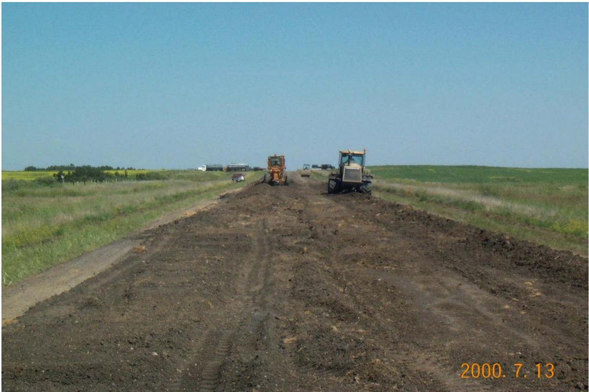
**Figure 11 – Blading, Water Spraying and Compaction Procedure**
