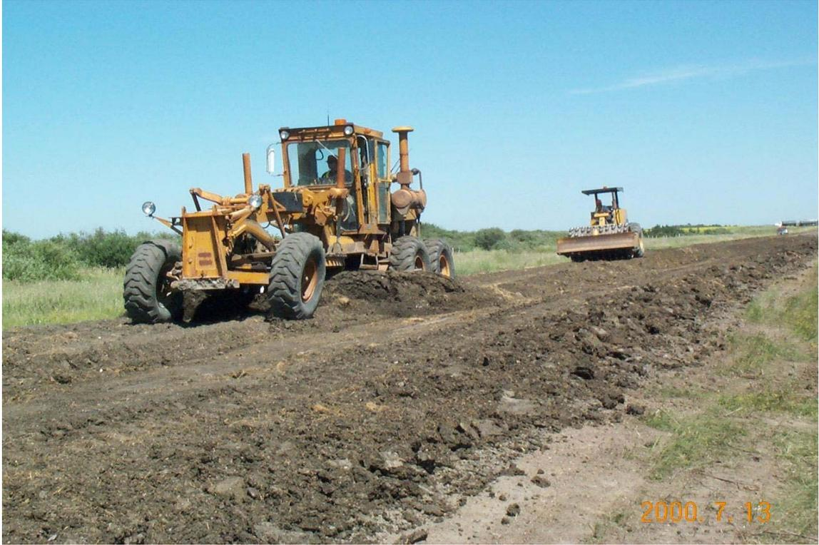
**Figure 10 – Blading Off Geocomposite**
