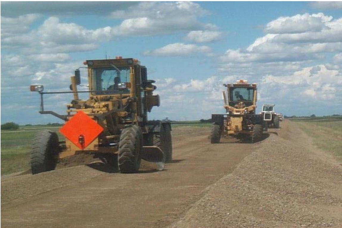
**Figure 13 – Base Aggregate Overlay**
