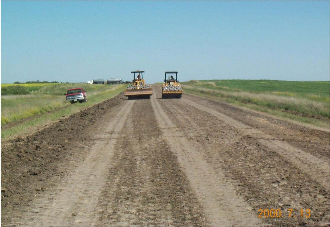
**Figure 12 – Road Compaction Procedure**
