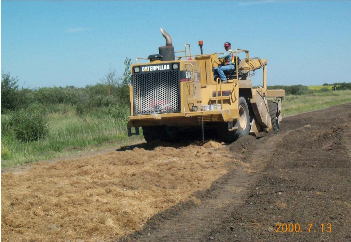
**Figure 8 – Rotomixing Flax Straw Into Subgrade**
