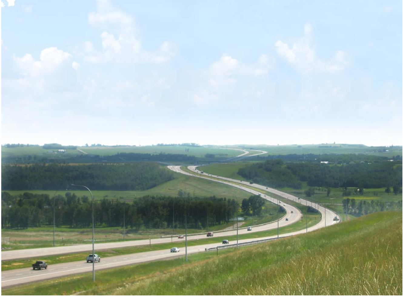
Figure 9: Photo of Deerfoot Trail Extension Crossing Bow River Valley
