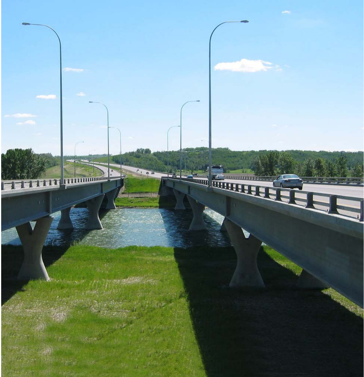
Figure 8: Photo of Bow River Bridges
