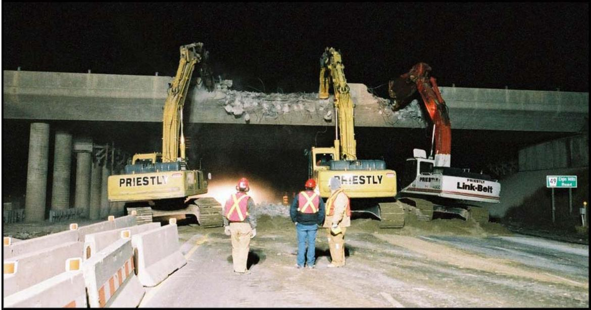
Figure 8 - Demolition commences with removal of parapet walls
