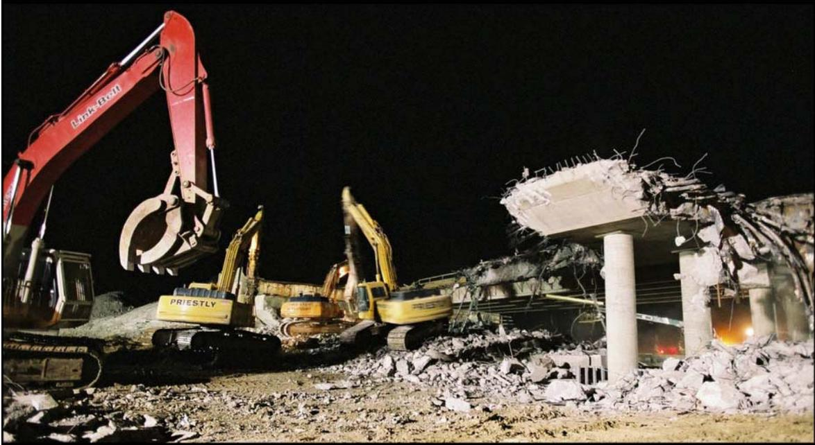
Figure 10 – Centre piers remain following deck removal on either side
