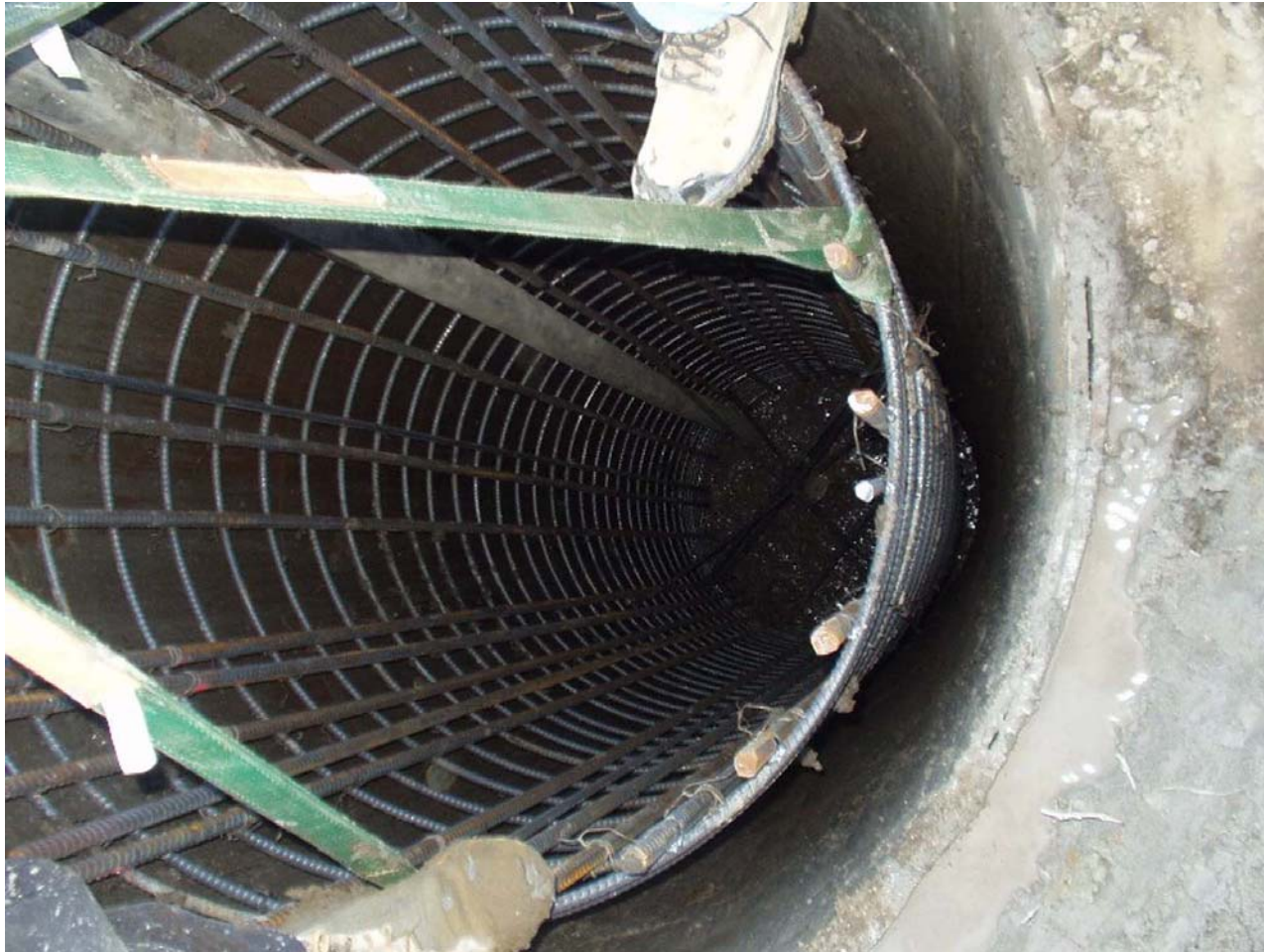
Figure 3: SCC is Being Poured into The Tangent Pile
