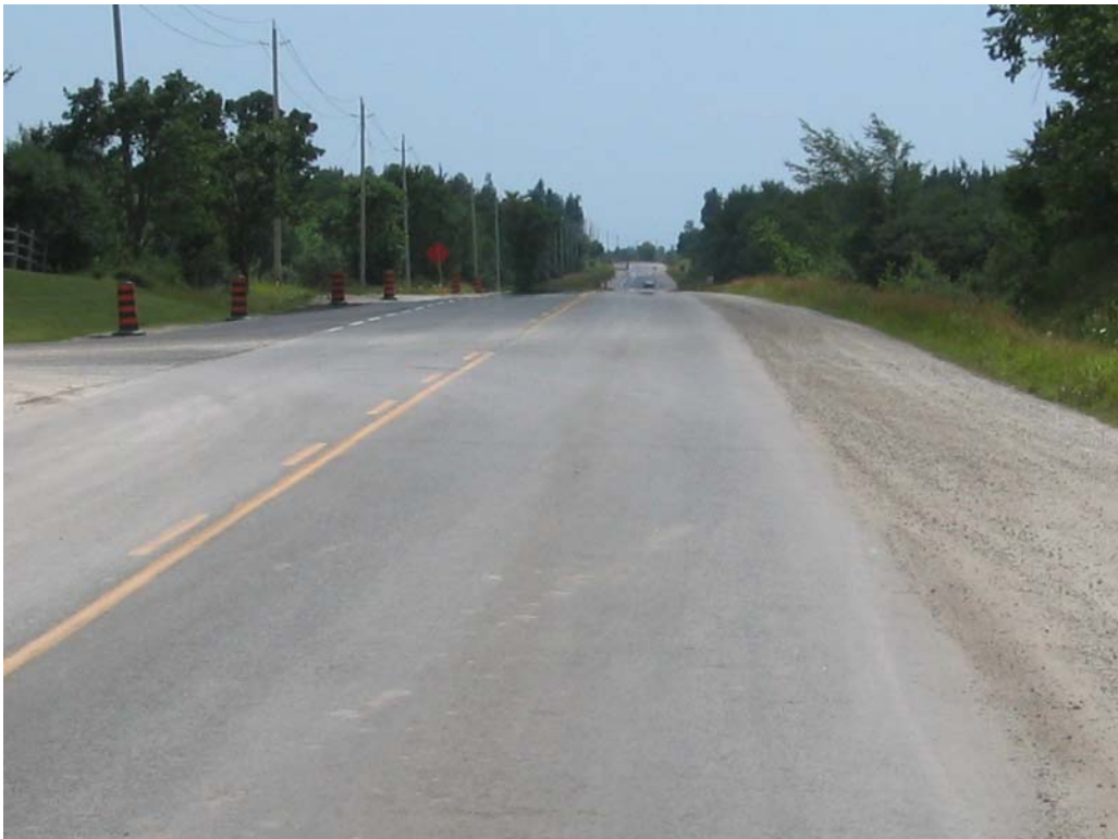
Figure 5. Completed Surface of Cold-In-Place Recycled with Expanded Asphalt mix.
