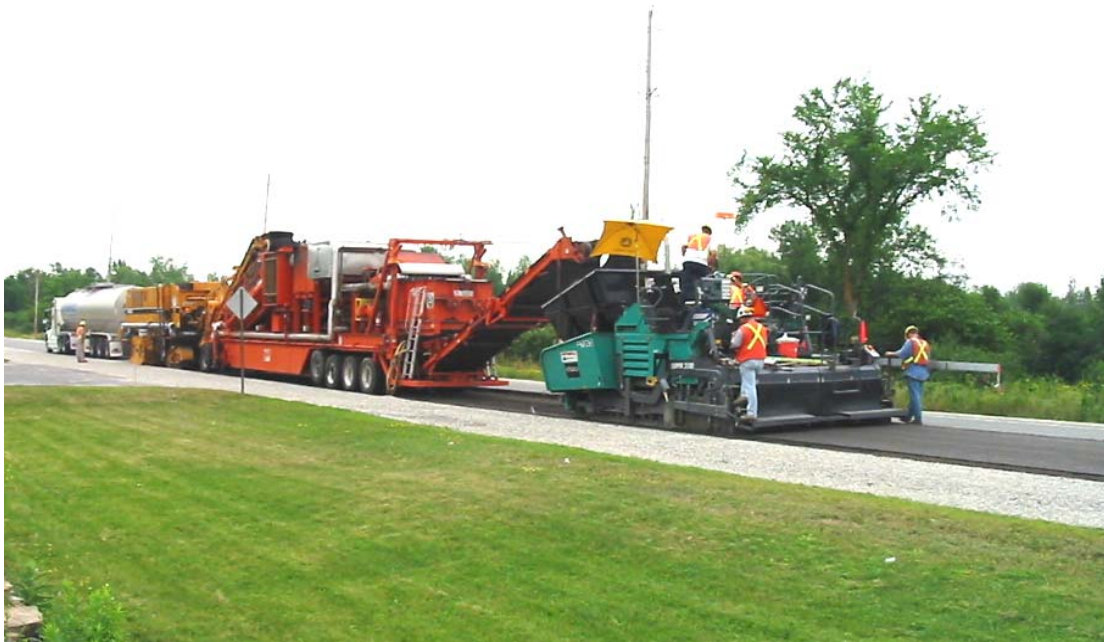
Figure 3. Cold-In-Place Recycling with Expanded Asphalt Train.
