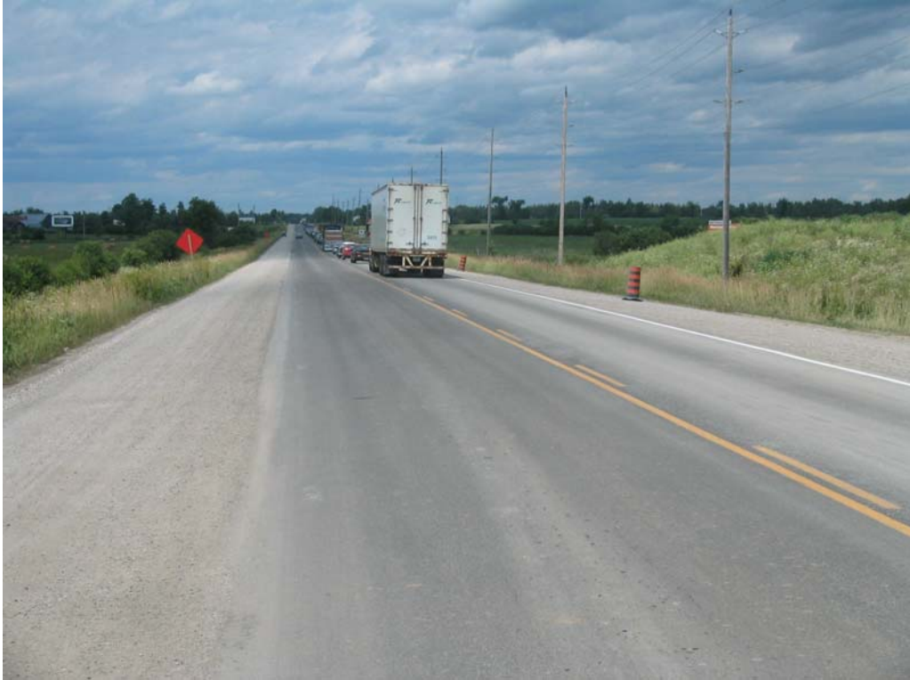
Figure 4. Completed Surface of Cold-In-Place Recycled mix.
