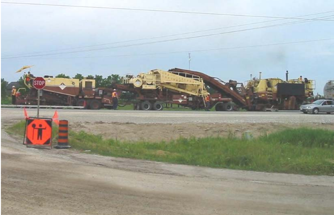
Figure 2. Cold-In-Place Recycling Train.
