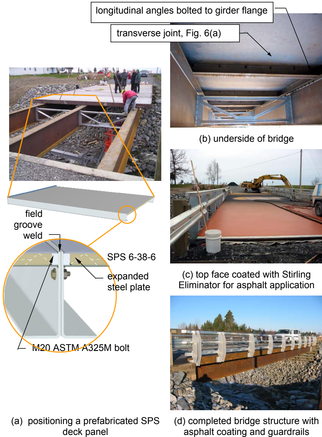
Figure 6 - Shenley Bridge Erection
