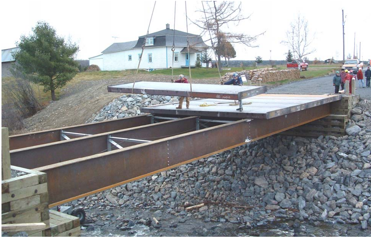
Fig. 4. Positioning one of ten Sandwich Plate System bridge deck panels
