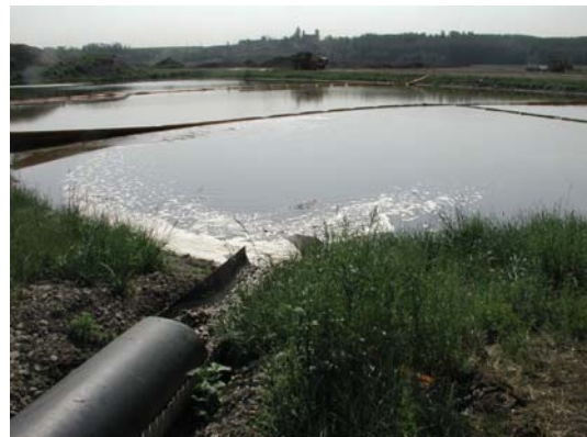
Wash water returned to settling ponds
