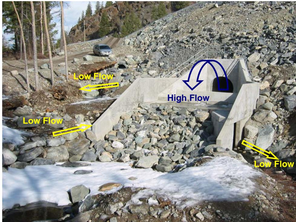
**PHOTO 2 – OVERFLOW OUTLET PROTECTION FOR SPAWNING CHANNEL**
