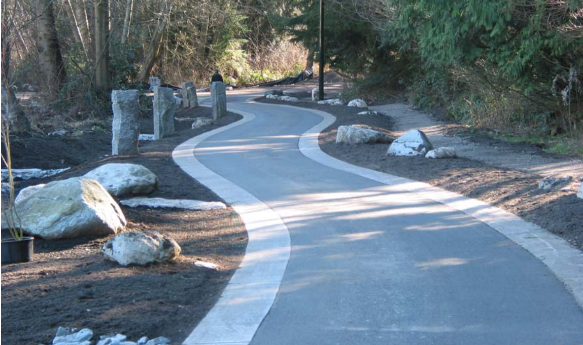
Figure 4: Narrowed Meandering Road Alignment - One Way Section
