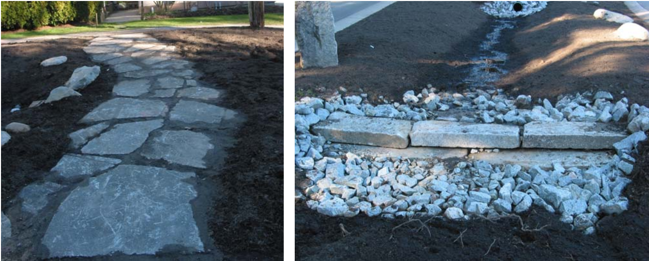
Figure 3: Recycled Concrete Walks and Recycled Granite Drop Structure
