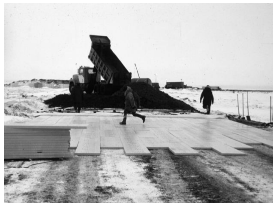
Figure 7 : Insulation installation (Courtesy of John Zarling)
