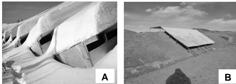
Figure 9 : Snowsheds in Bonanza Creek, Alaska (A) and Sunsheds, Qinghai-Tibet Roadway (B) (Courtesy of John Zarling (A) and of Professor Ma, Lanzhou, China (B))
