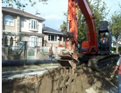
Sheep's-foot roller with soil reuse
