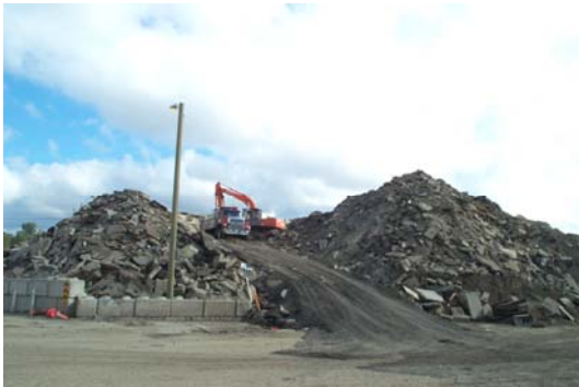
Crushing Operation from Stockpile to Finished Road Base Product
