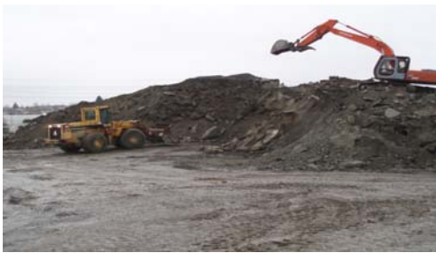
Typical Excavated Waste Stockpile
