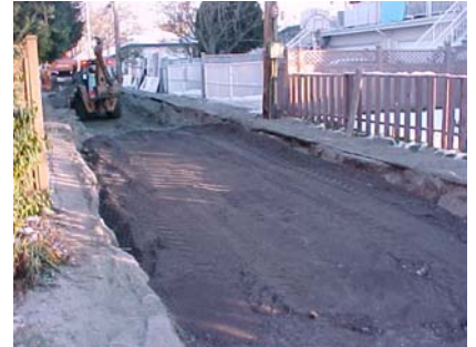
Sub-base of blended material
