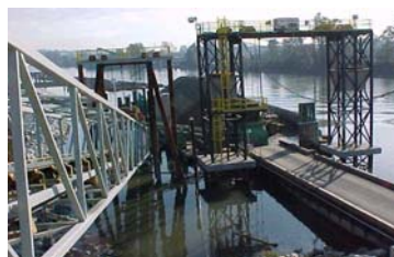
Barge Unloading Facility
