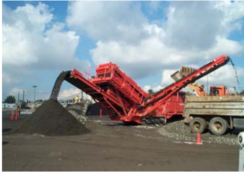
Screening and Blending of Excavated Soil
