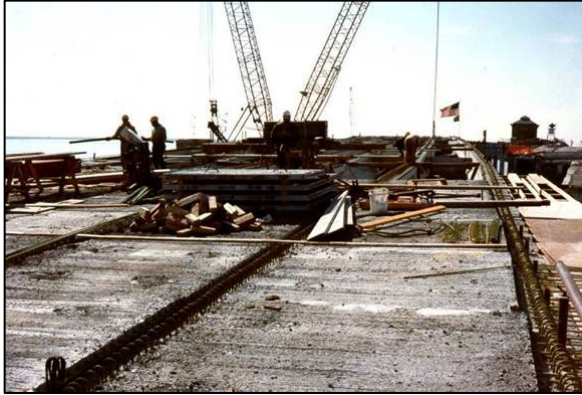
Precast deck slab placement
