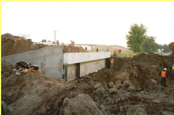
First abutment in place
