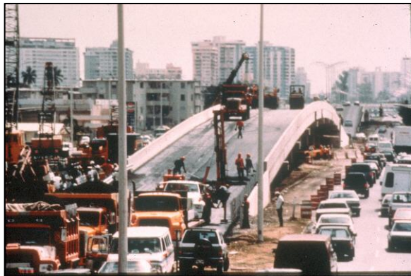
Membrane and asphalt wearing surface
