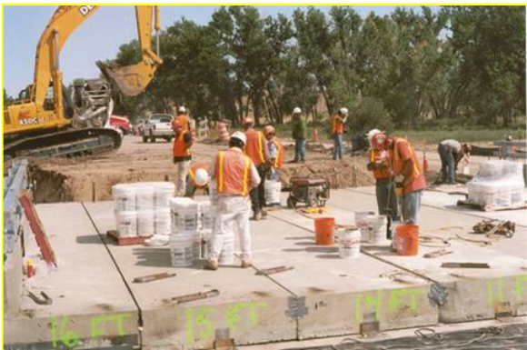
Grouting the deck joints
