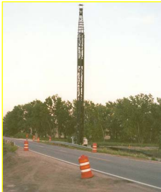
Pile driving in advance
