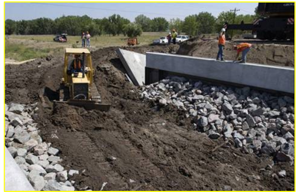
Grading and riprap under bridge
