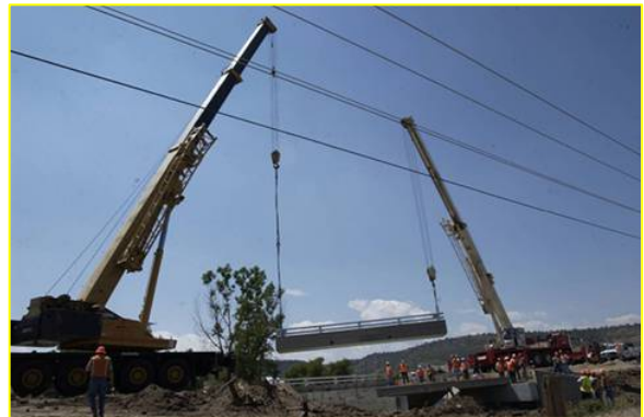
Install precast superstructure slabs
