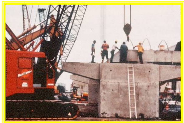
Precast pier cap installation
