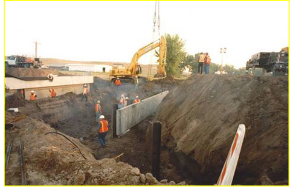
Stream work begins
