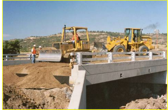
Backfilling & road approach work
