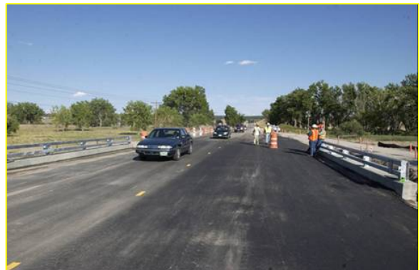
New bridge is open for traffic
