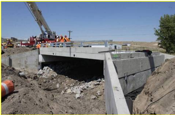
The completed structure
