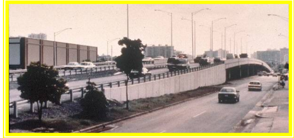
Completed bridges with traffic
