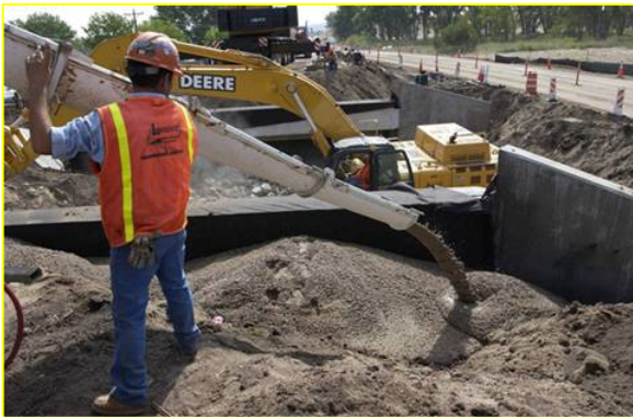
Flow-filling behind abutments
