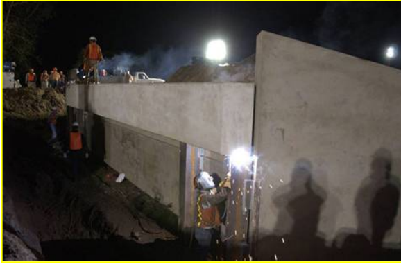
Weld substructure units together
