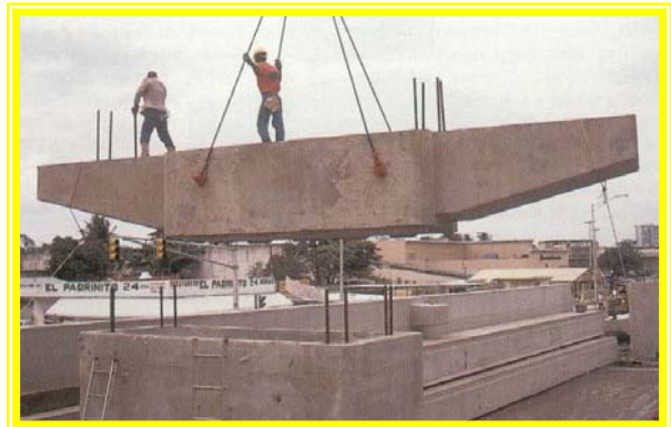
Precast pier cap installation
