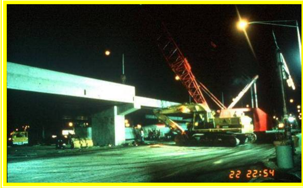
Adjacent box beam installation
