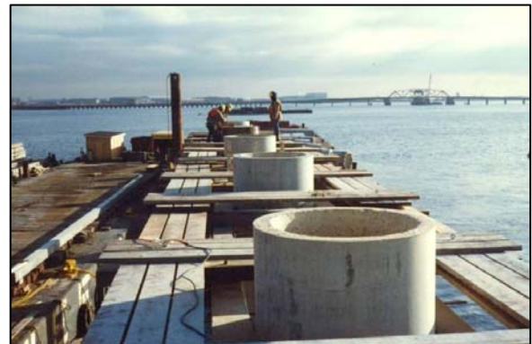
Precast cylinder piles
