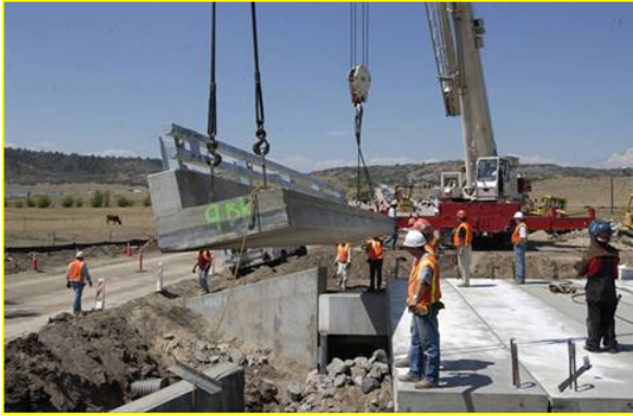
Placing edge girder - integral curb & rail
