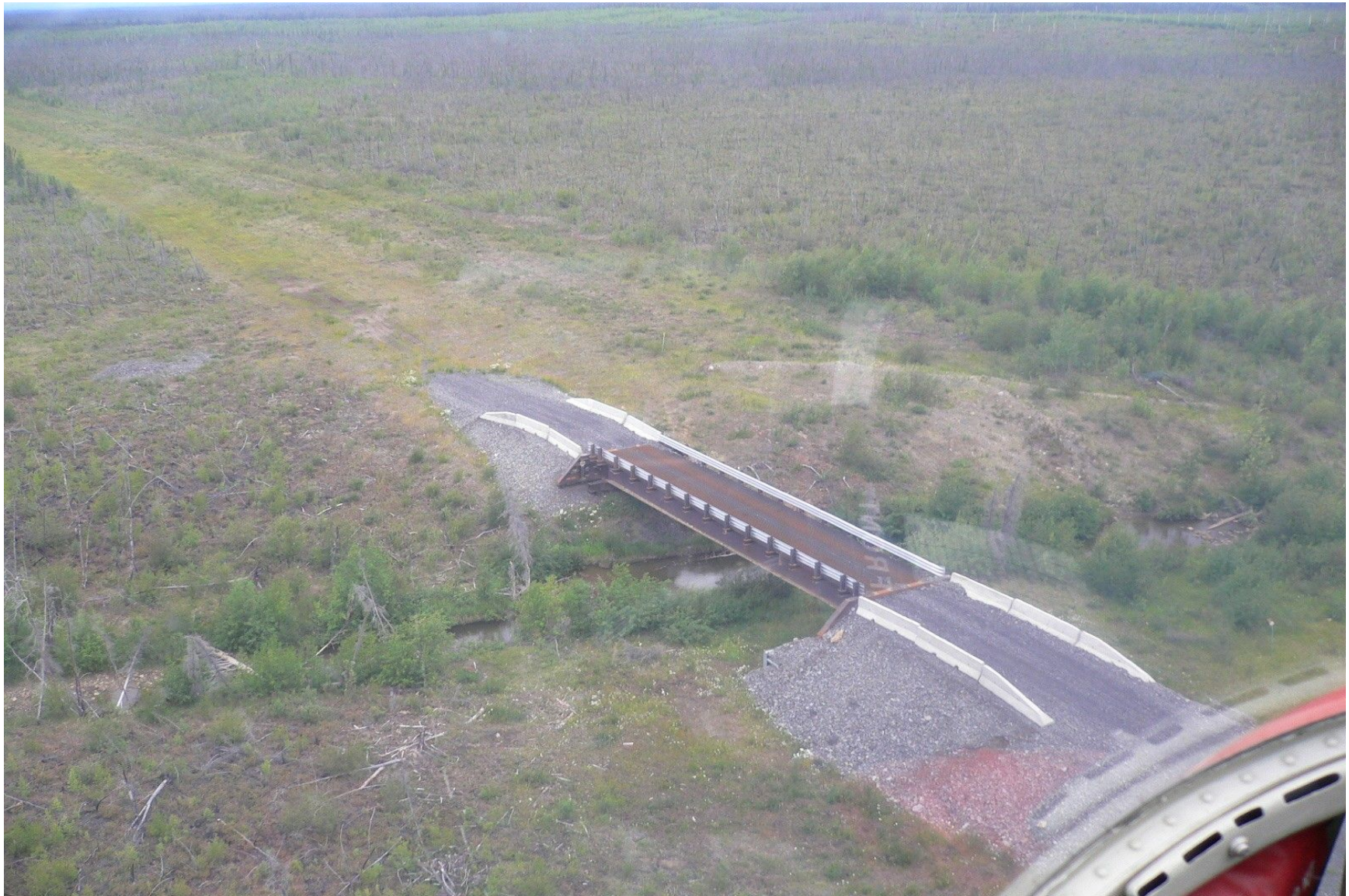
Figure 5: Notta Creek Bridge at 982.3km
