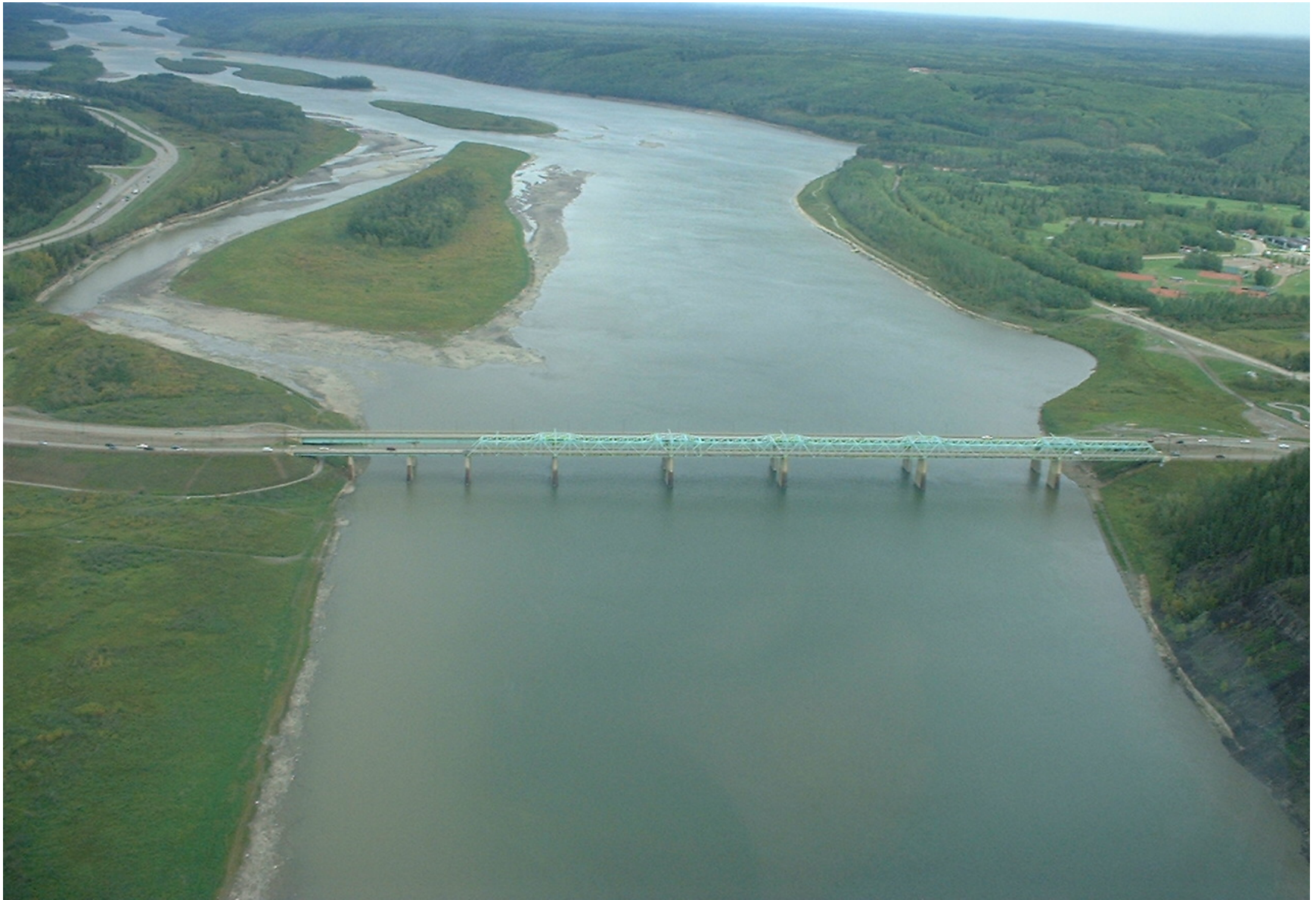
Figure 4: Aerial Photo of Grant MacEwan Bridge over Athabasca River in Fort McMurray
