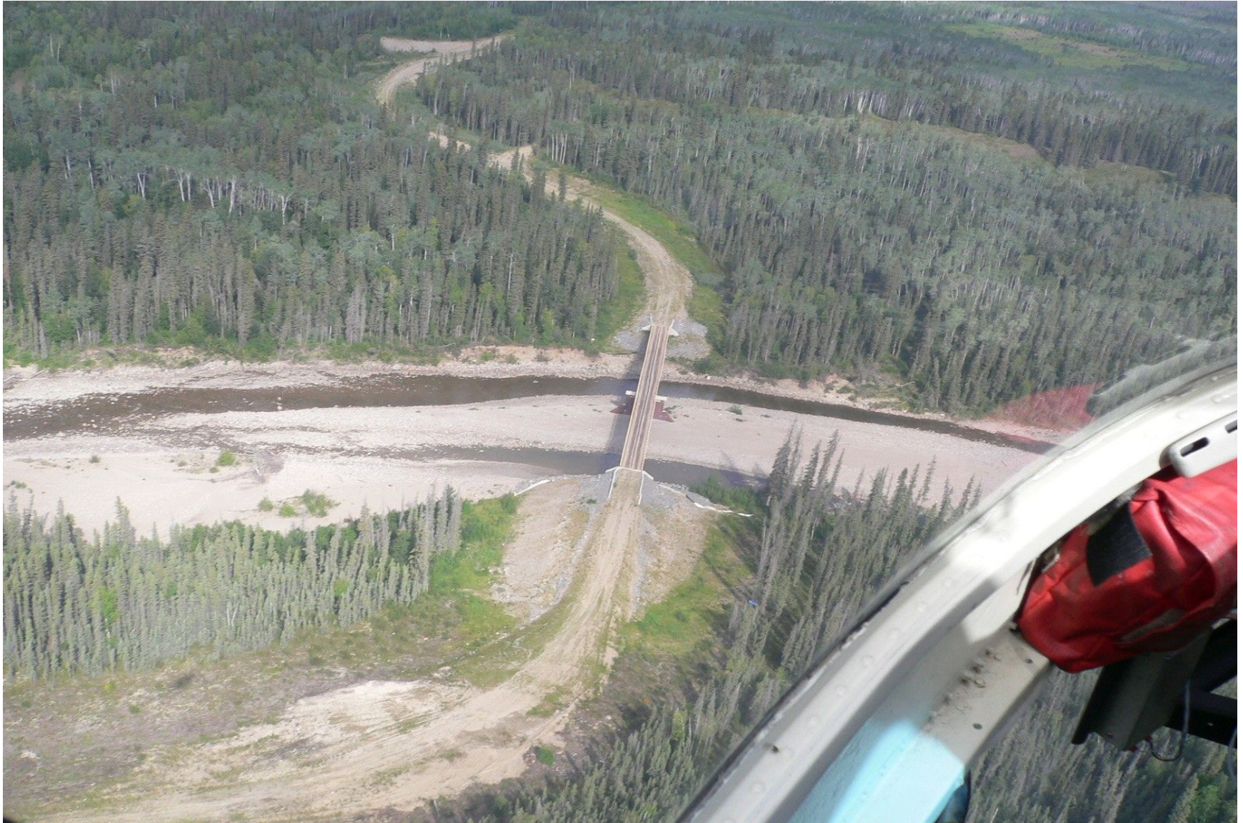
Figure 6: Ochre River Bridge at km 722.4
