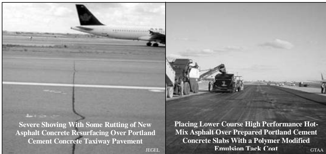
Photograph 7. Localized Severe Shoving of New Asphalt Concrete Resurfacings of Some Heavy Aircraft Traffic Areas at Pearson International Airport in Toronto Has Required the Development of High Performance Hot-Mix Asphalts and Special Construction Methods Such as Polymer Modified Emulsion Tack Coats
