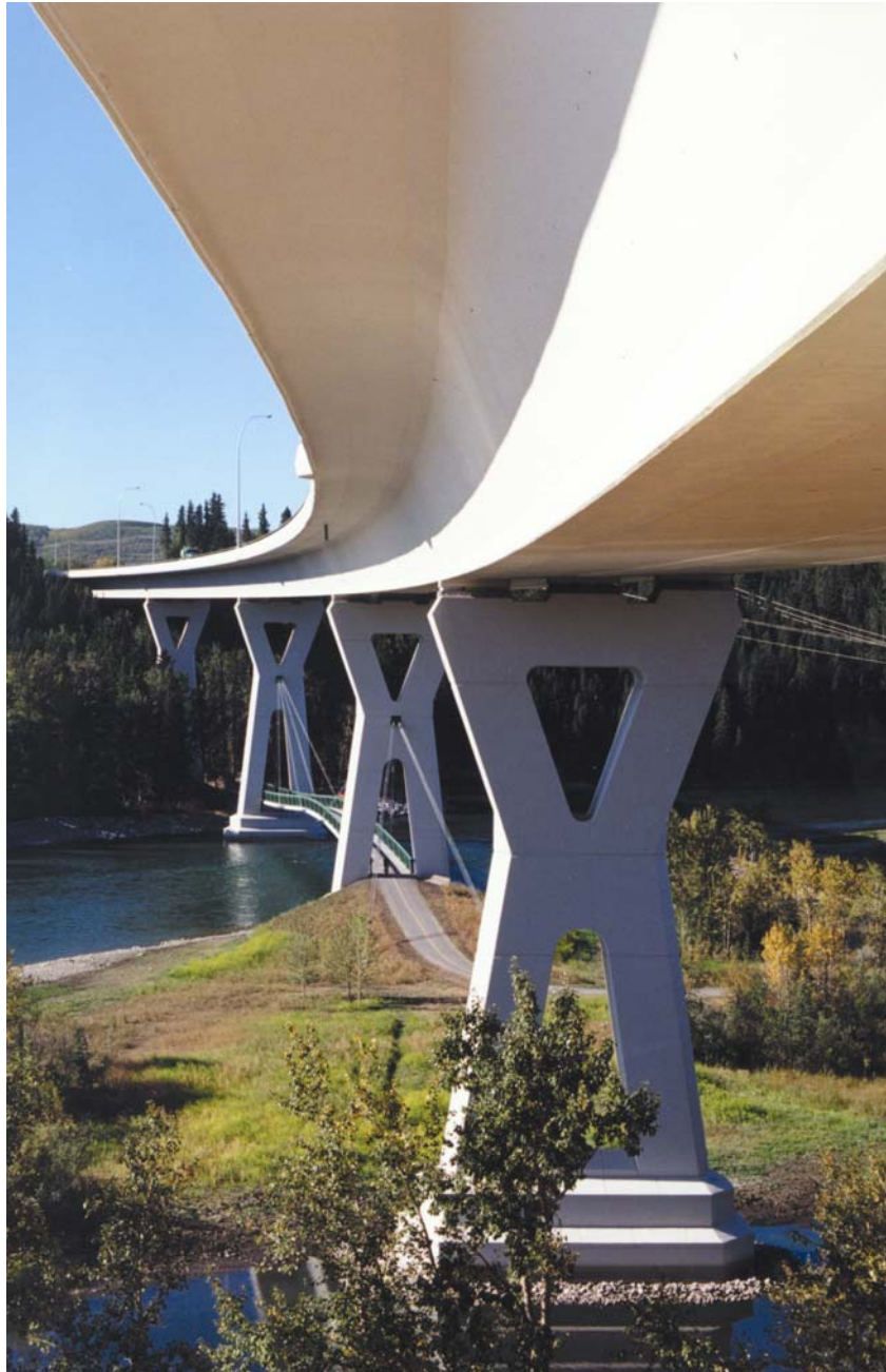
Photo XXII – Stoney Trail Bridge Over Bow River
