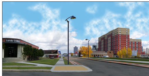
3. New Sidewalks, Curbs and Light Standards
