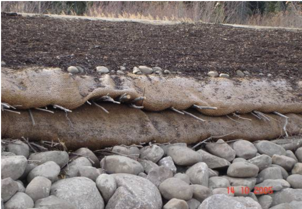
Photo 7 Vegetated Mechanically Stabilized Earth
