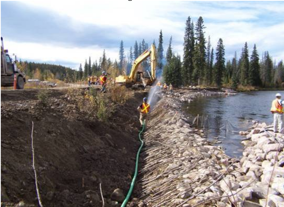
Photo 5 Live Siltation Implementation
