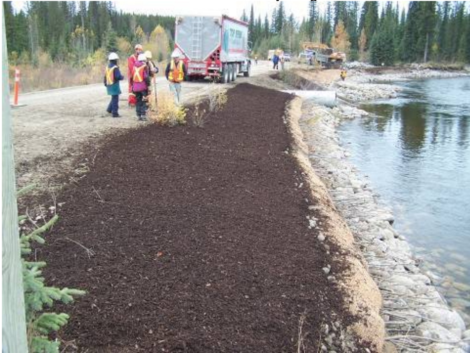
Photo 9 Sprayed compost blanket
