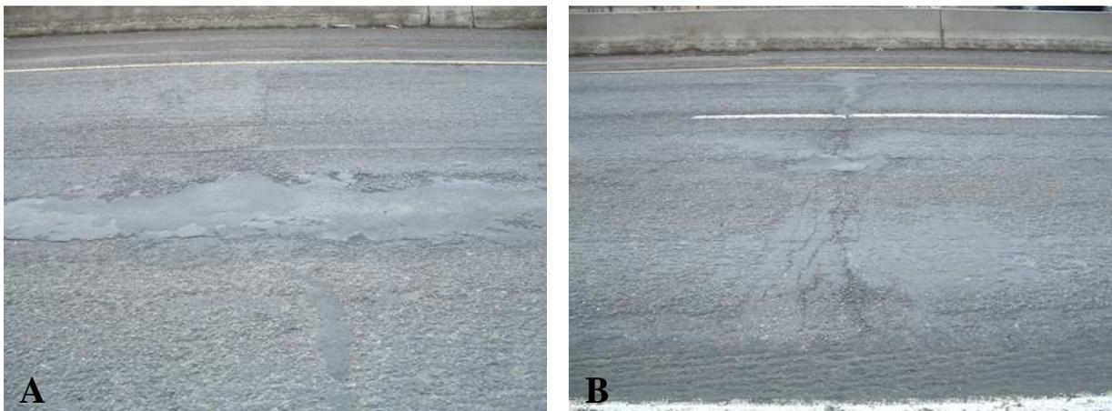
Figure 3 – Examples of QEW Condition: A) Patching of Lane 2, B) Moderate Transverse Cracking
