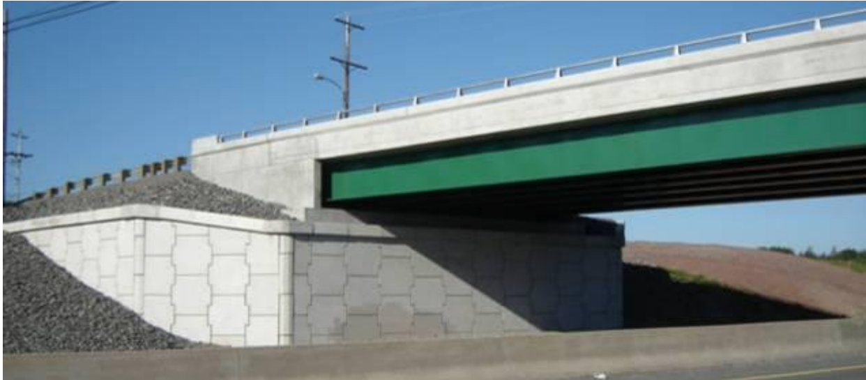
Figure 11 – New Coxheath Road Bridge
