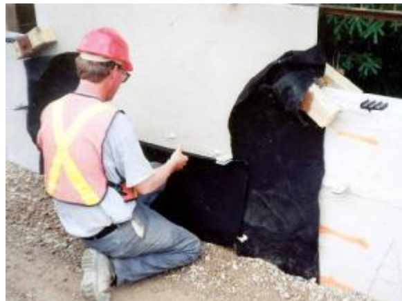
Figure 12 – Geotextile on Rear Face Joint
