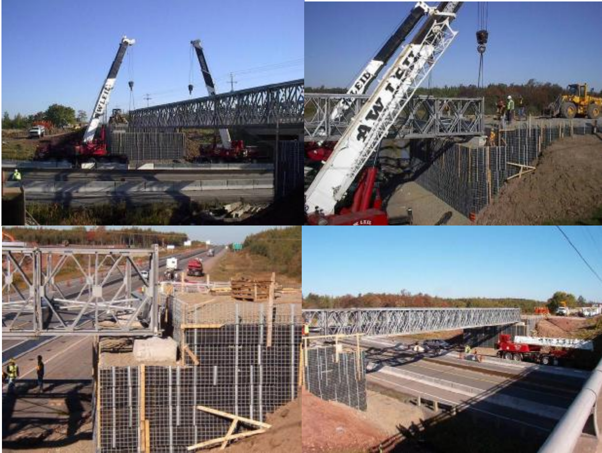
Figures 16 to 23 - Modular Truss Bridge Erection Sequence
