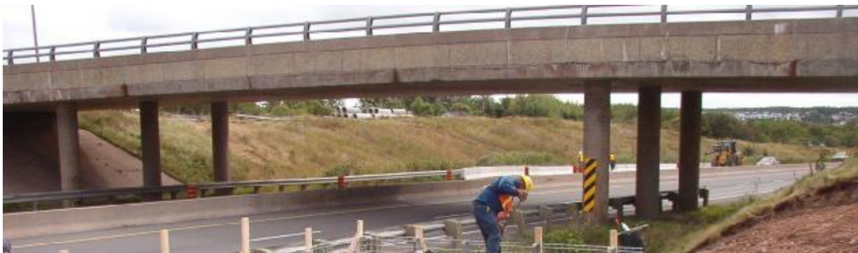
Figure 10 – Existing Coxheath Road Bridge
