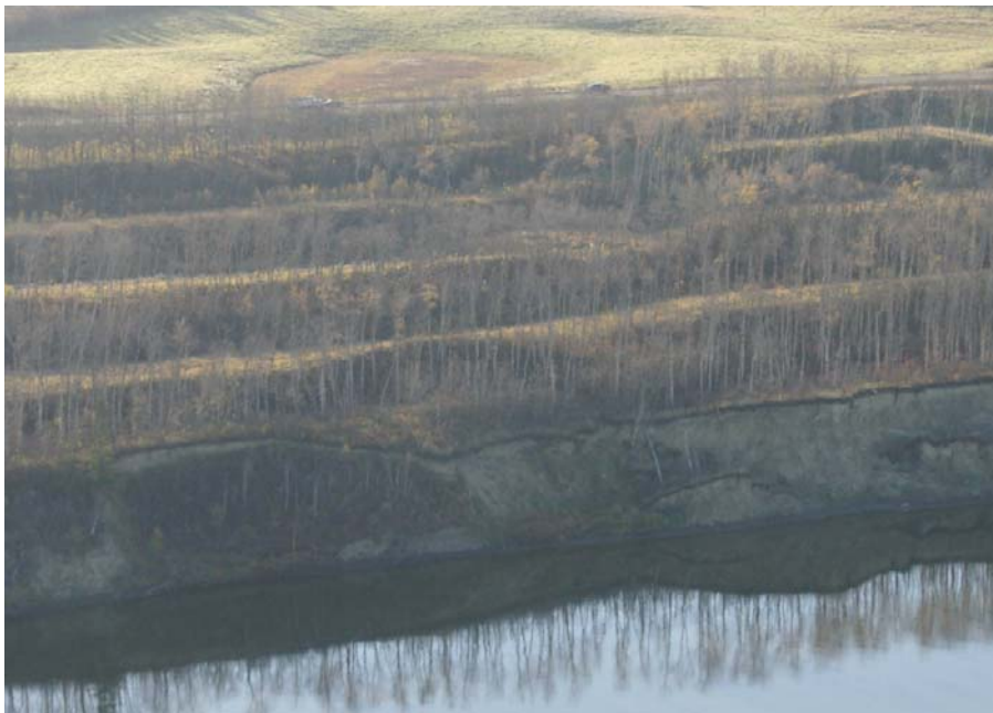
Figure 2. Photograph showing multiple landslide blocks.
