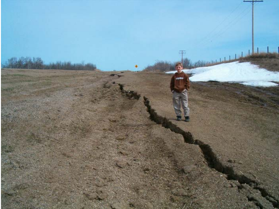
Figure 3: Landslide head scarp in upslope highway ditch (Photo taken on 16 April 2006).
