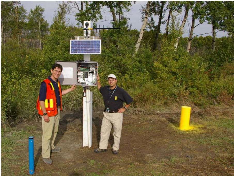
Figure 5. Photograph showing instrumentation nest near the highways
