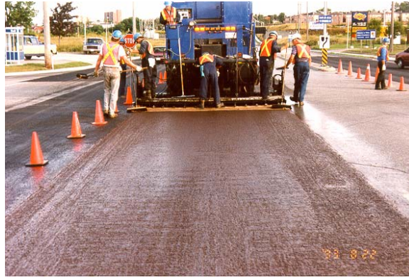
Figure 3 – Rut filling with microsurfacing lower lift on Thickson Road in Whitby, Ontario in 1993.
