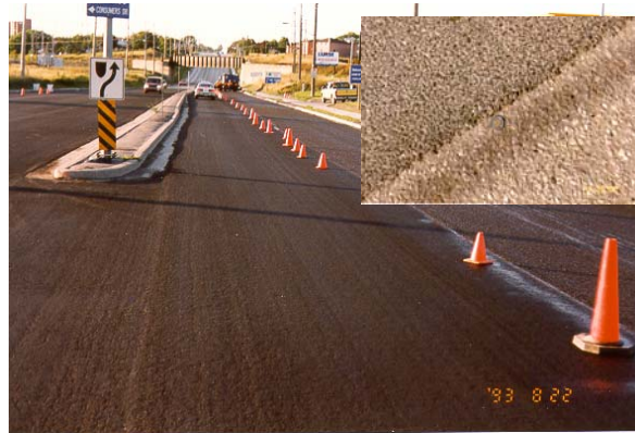
Figure 4 – Application of the second lift of microsurfacing.
