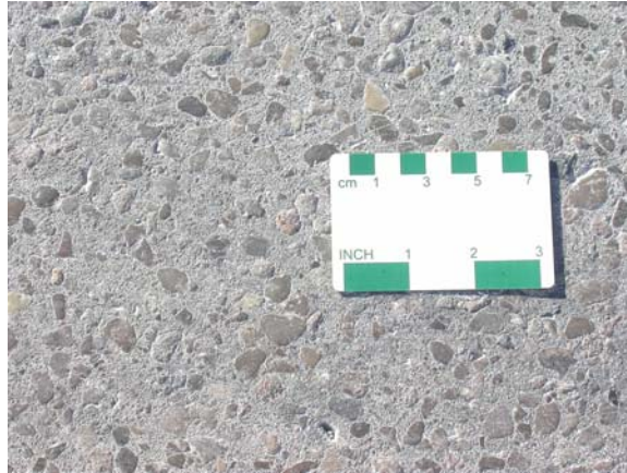
Figure 2 – Close up of pavement surface texture on before microsurfacing application.
