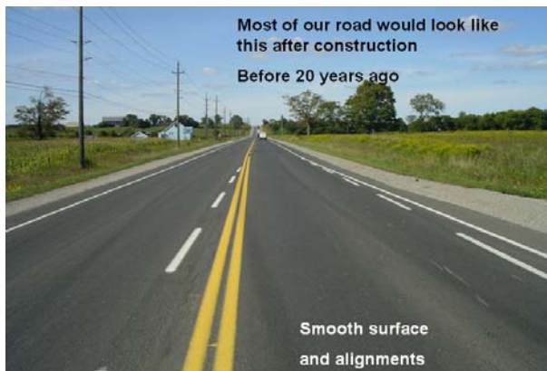
A newly constructed arterial 20 years ago
