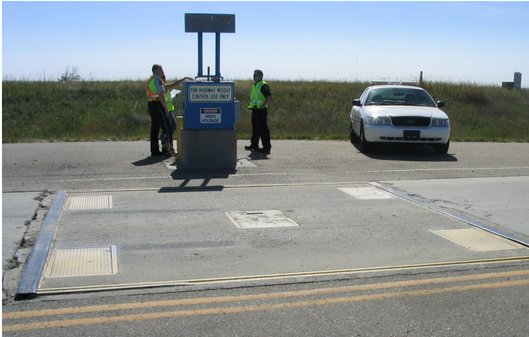
Figure 1: Existing static scale at Macklin enforcement site
