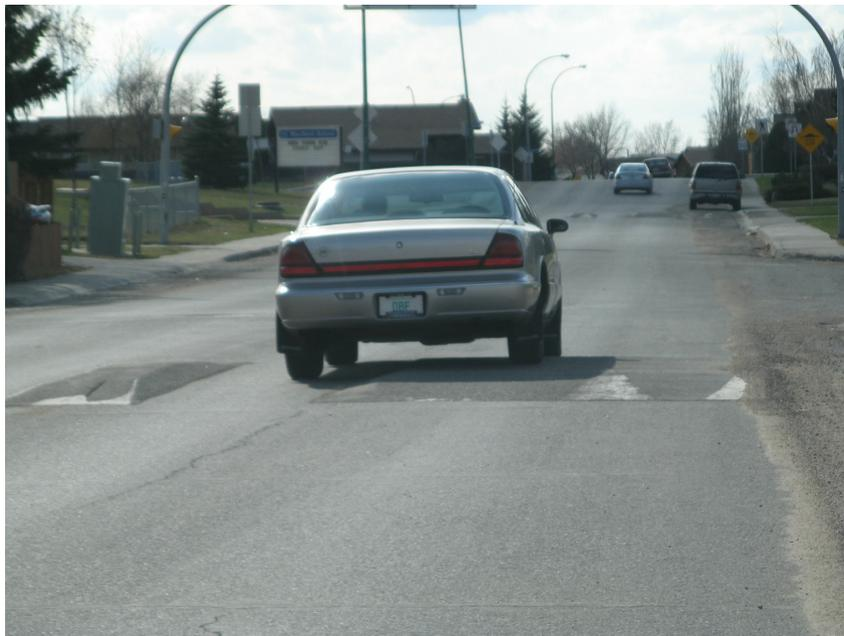
Figure 12 – Proper Use of Speed Cushion – Dry Conditions
