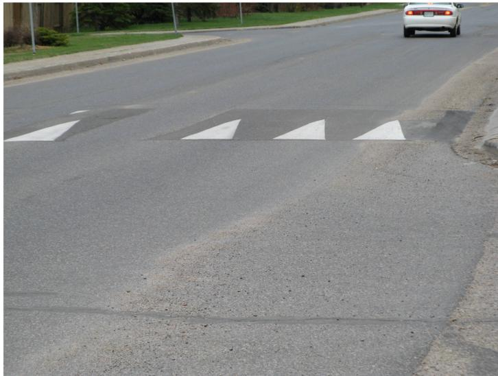
Figure 10 – Speed Cushion During Dry Conditions – Alternate View
