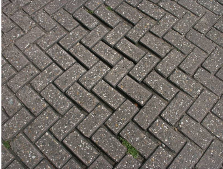
Figure 6. High Severity Excessive Joint Width. (greater than 10 mm with loss of joint sand and misalignment)
