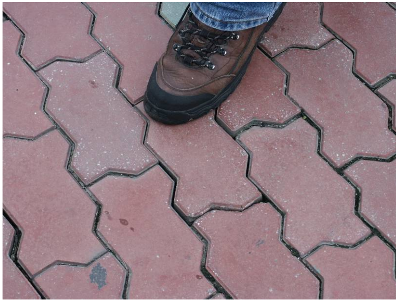
Figure 4. Low Severity Excessive Joint Width. (less than 6 mm wide with or without joint sand loss and performing well)
