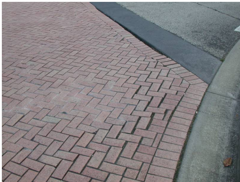
Figure 5. Medium Severity Excessive Joint Width.
