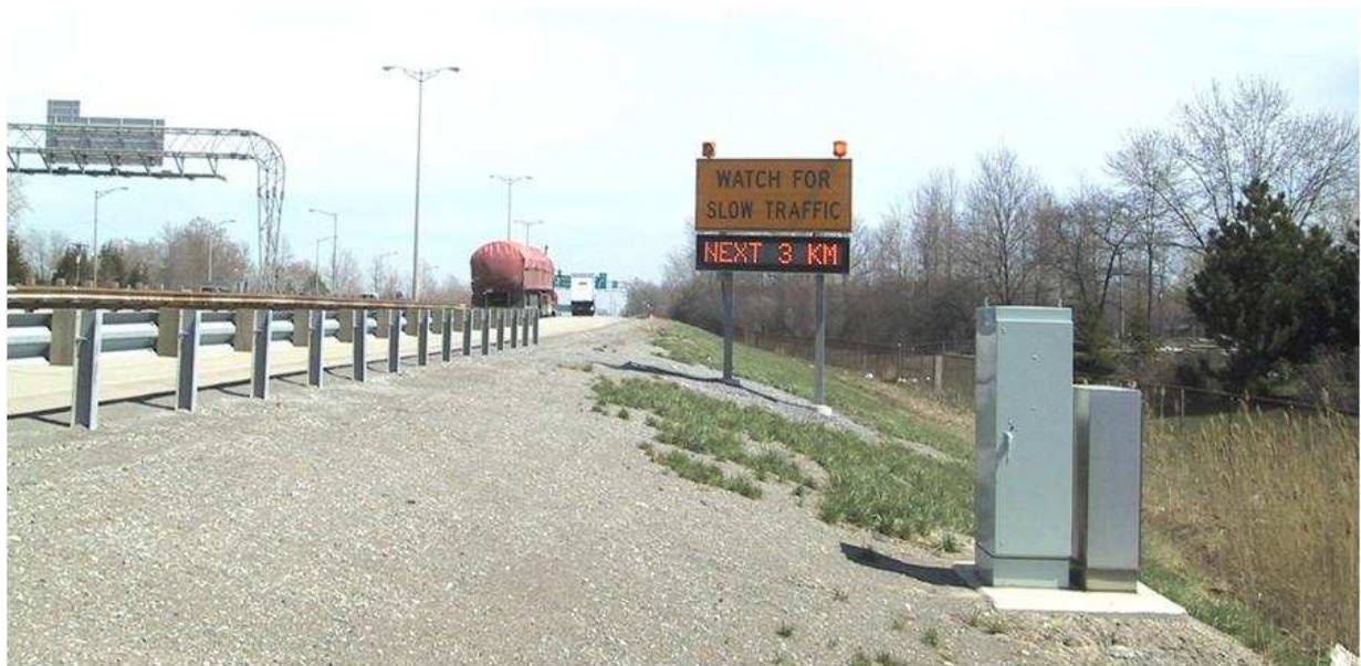
Figure 3 Typical QWS Cabinet and Warning Sign Site Installation
