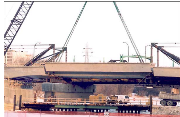
Provencer Bridge, Winnipeg, MB [16]
