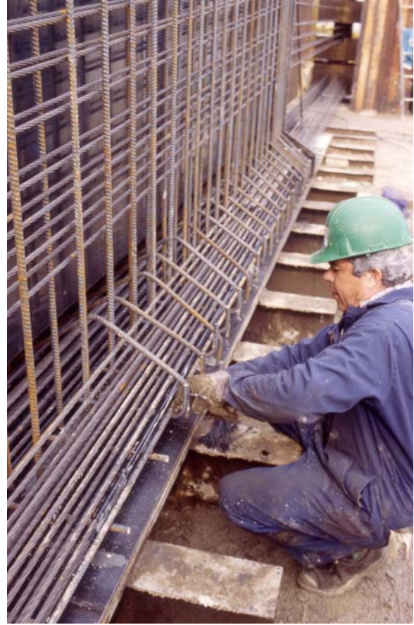
Conventional rebar reinforcement
