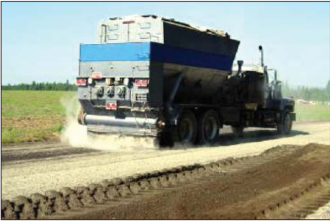
Figure 7 – Placing cement dry.
