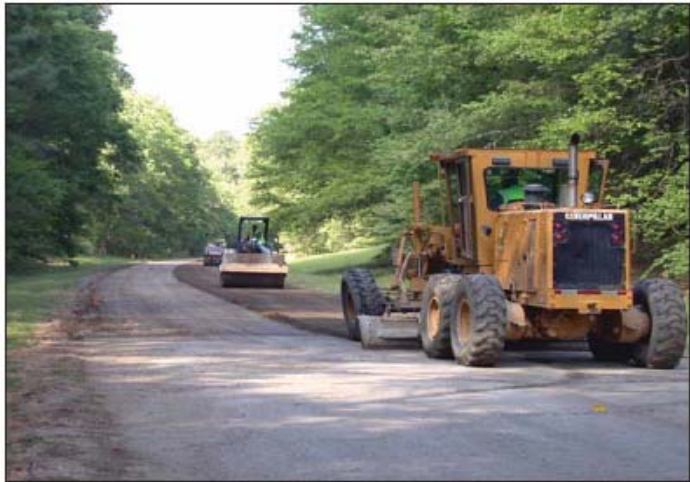
Figure 10 – Compaction and final grading.
