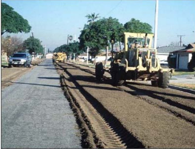
Figure 6 – Grading and shaping.
