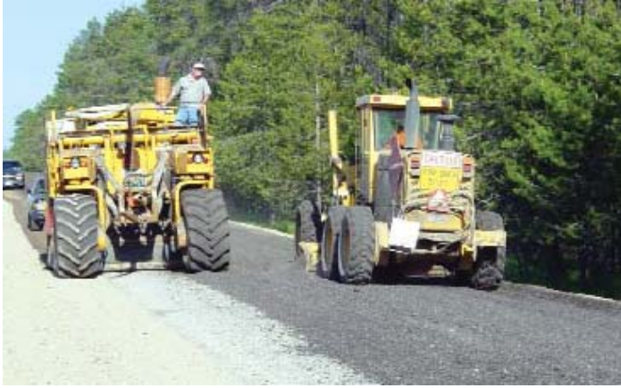
Figure 12 – Pulverizing and grading operations in Spokane County, Washington.
