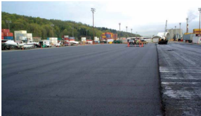
Figure 11 – New pavement next to curing FDR at Terminal 115 in Seattle, Washington.
