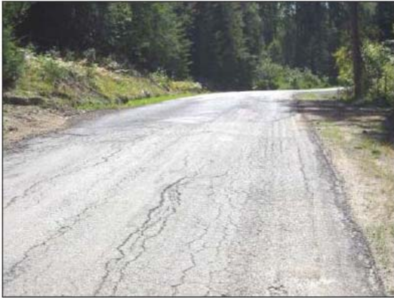
Figure 1 – Example of pavement distress indicating base problems.
