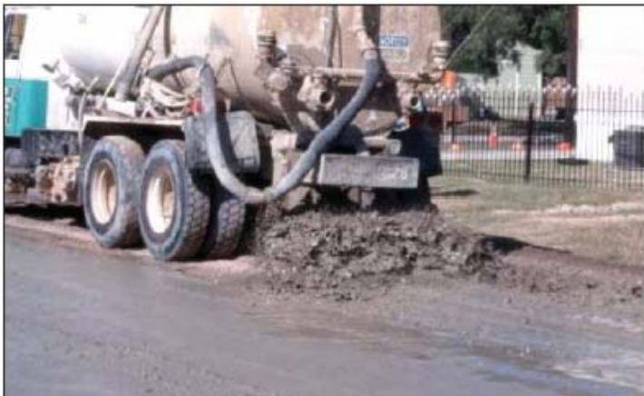
Figure 8 – Placing cement in slurry form.
