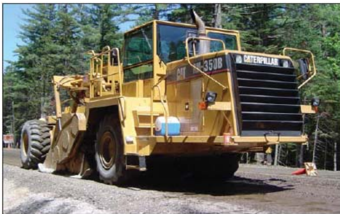
Figure 5 – Pulverizing a failed asphalt pavement.
