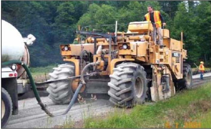
Figure 9 – Water being injected during mixing operation.
