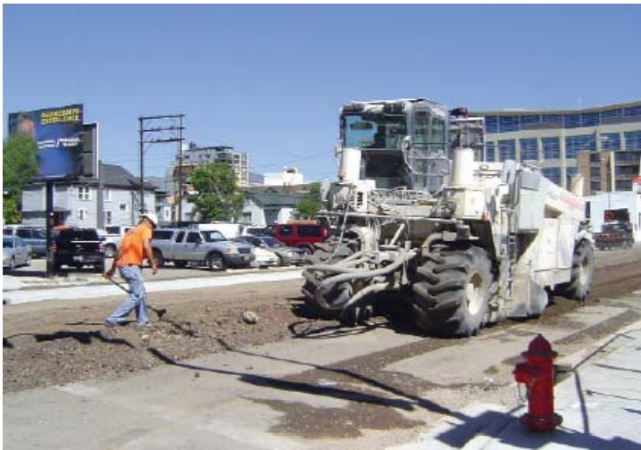
Figure 13 – Pulverizing failed flexible pavement in downtown Reno, Nevada.
