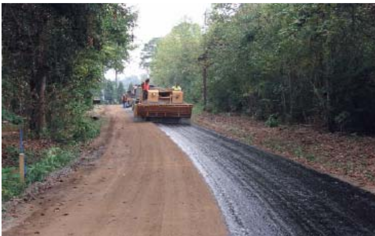
Figure 14 – Application of bituminous surface treatment in Fairfield County, South Carolina.
