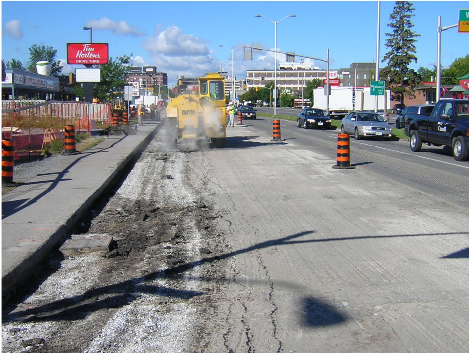
Figure 7: Rubblizer in Action on Carling Avenue
