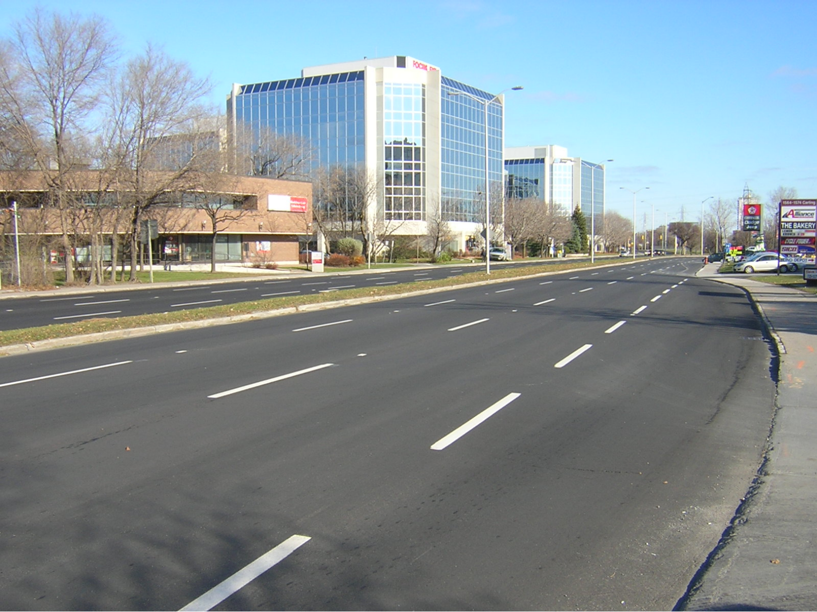
Figure 12: Completed Project - Carling Avenue with Superpave Asphalt on Rubblized Concrete Layer
