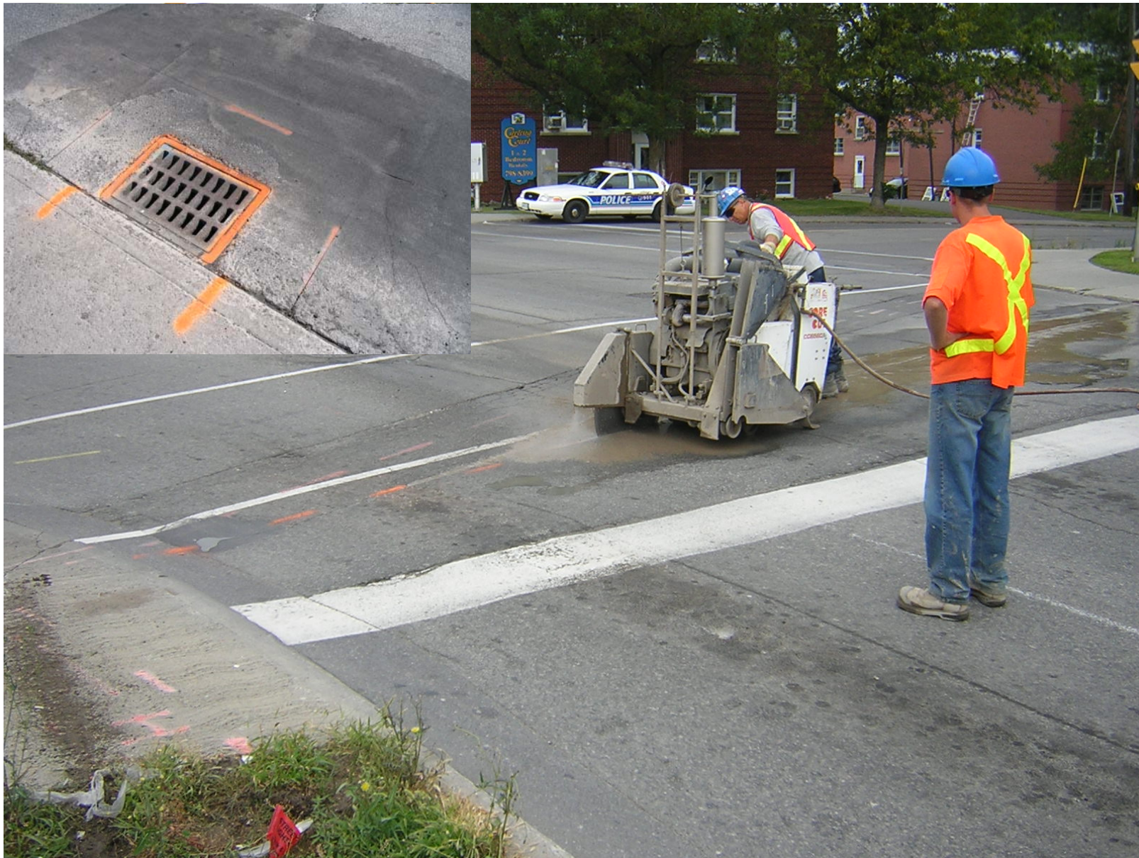
Figure 11: Saw Cutting to Separate Curbs, Intersections, Catchbasins and Manholes
