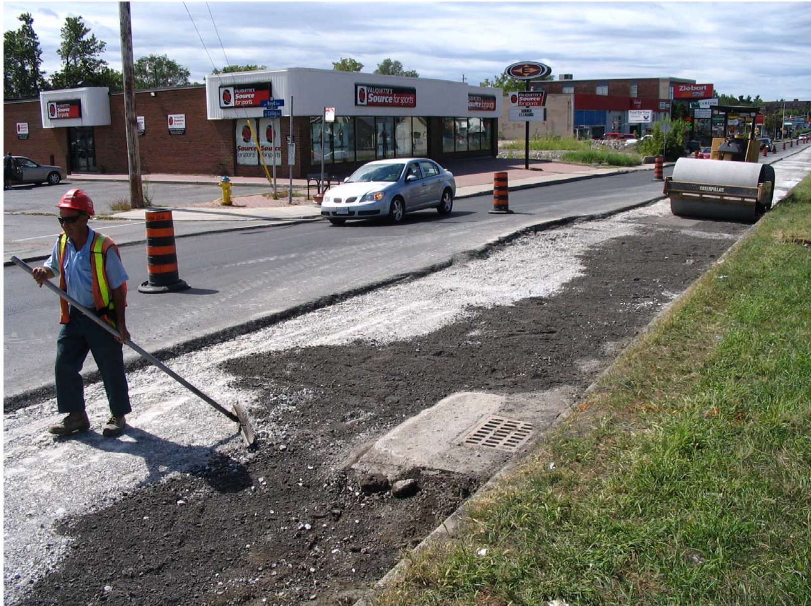
Figure 10: Levelling the Grade and Profile with Granular A and Compacting the Rubblized Surface
