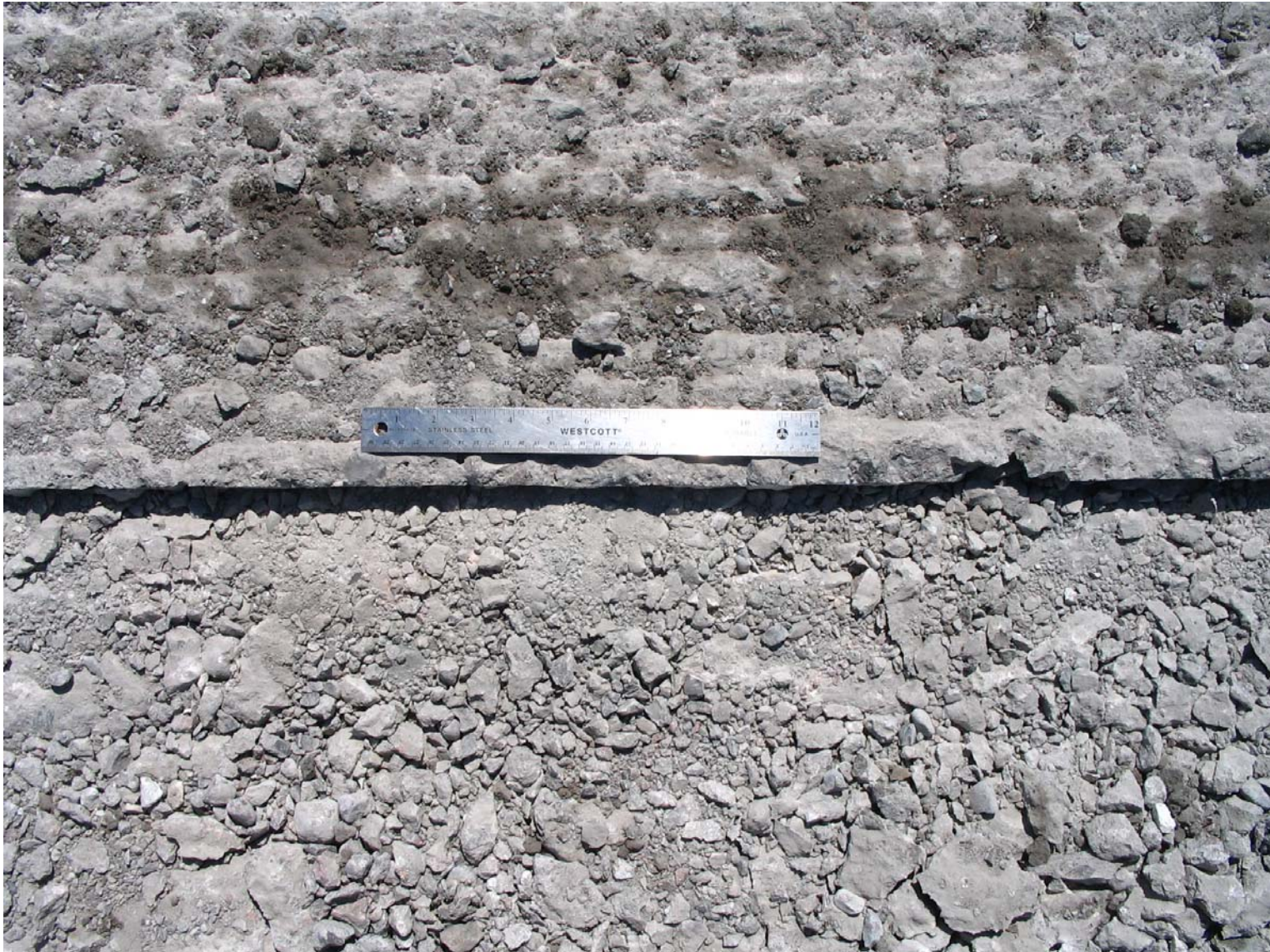
Figure 8: Comparison of Intact and Rubblized Concrete Surface (Plan View)
