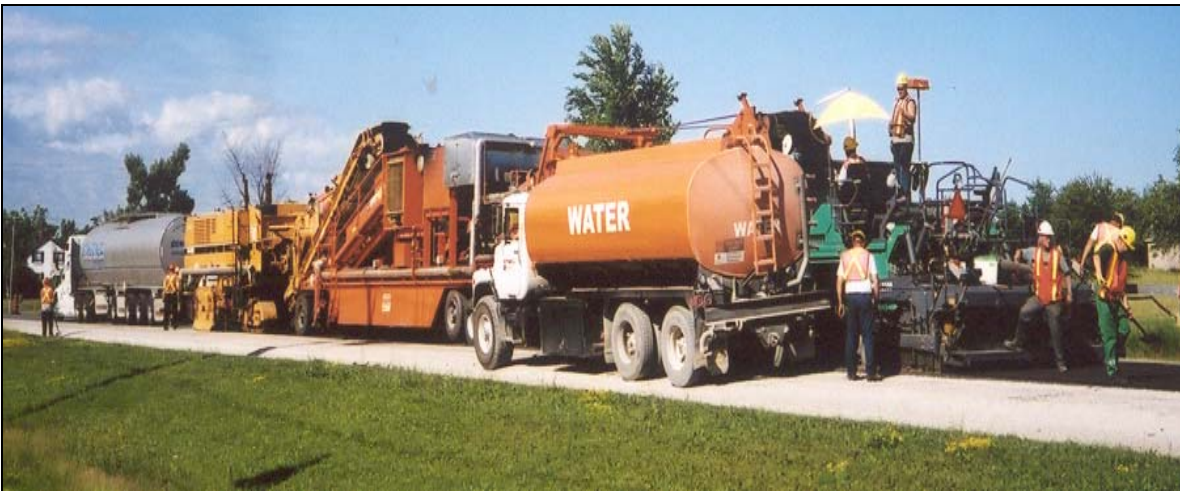
Figure 2. Cold-In-Place Recycled Expanded Asphalt Train
