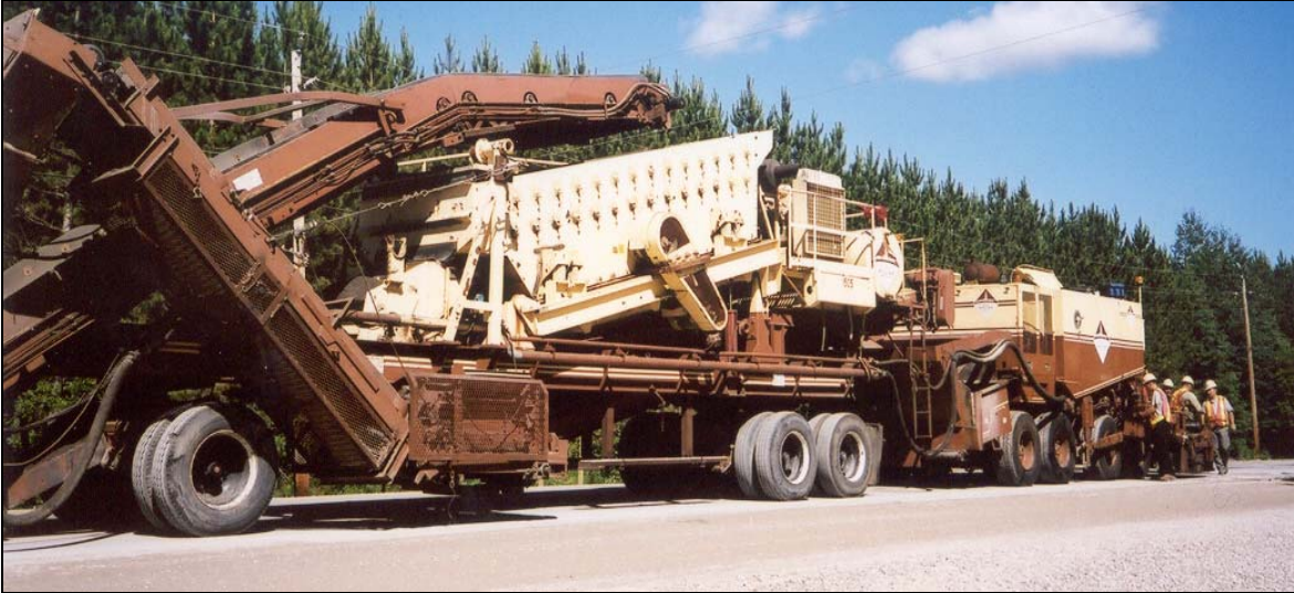
Figure 1. Cold-In-Place Recycling Train
