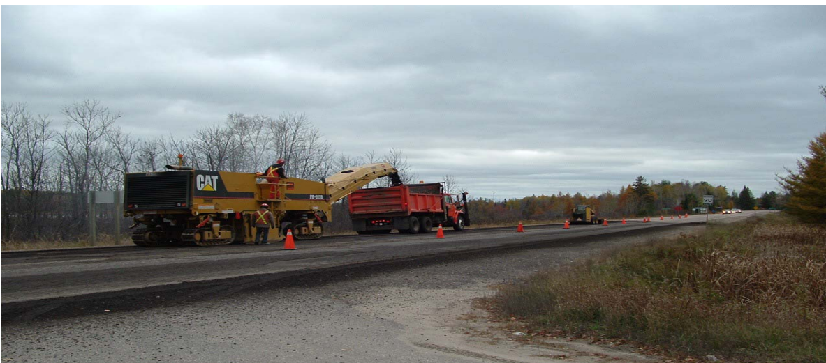
Figure 3. Traditional milling operation with HMA to follow
