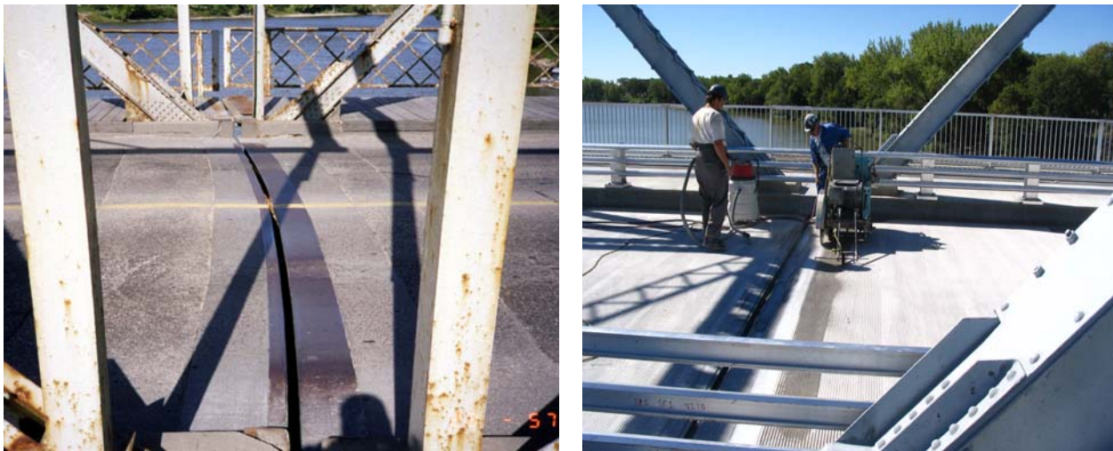
Figure 3. Replacing expansion joints
