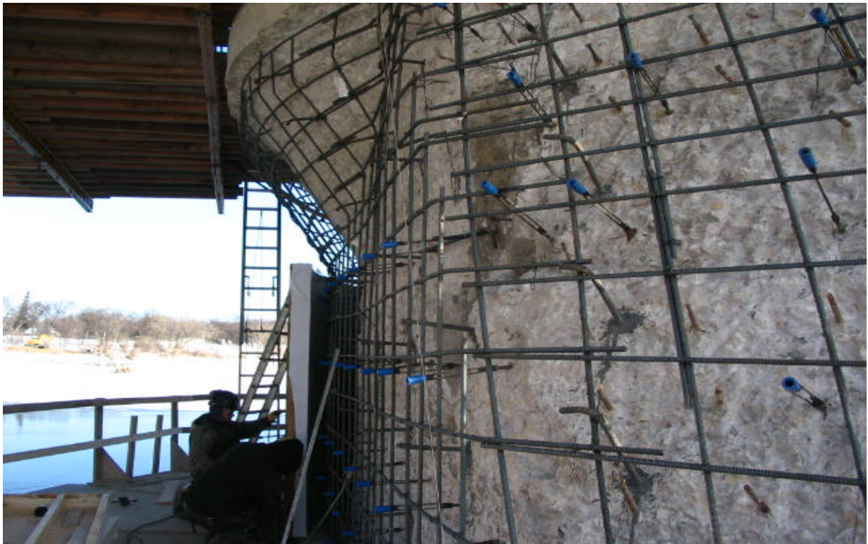
Figure 2. The pier concrete encasement reinforcing cage
