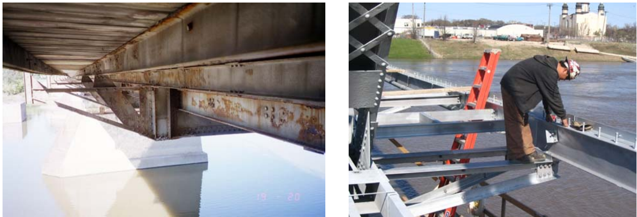
Figure 6. Existing and new sidewalk support brackets
