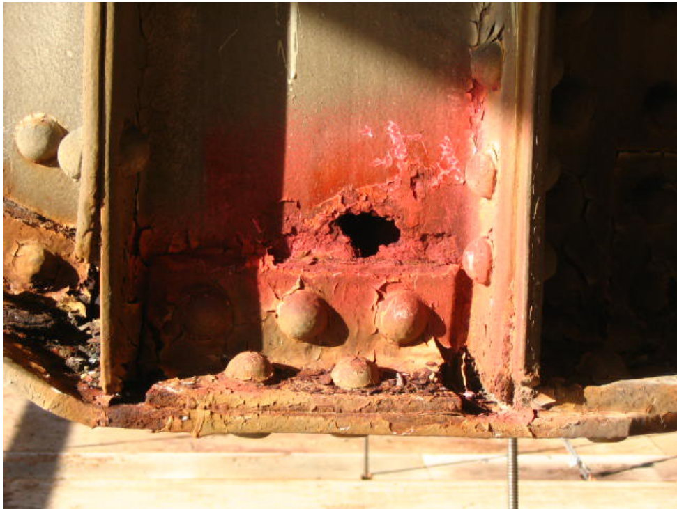
Figure 4. Bottom truss vertical member rusted through
