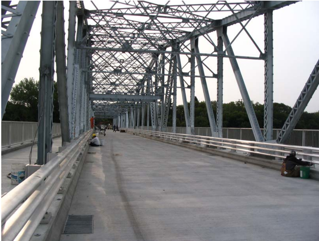
Figure 7. Bridge traffic railing system
