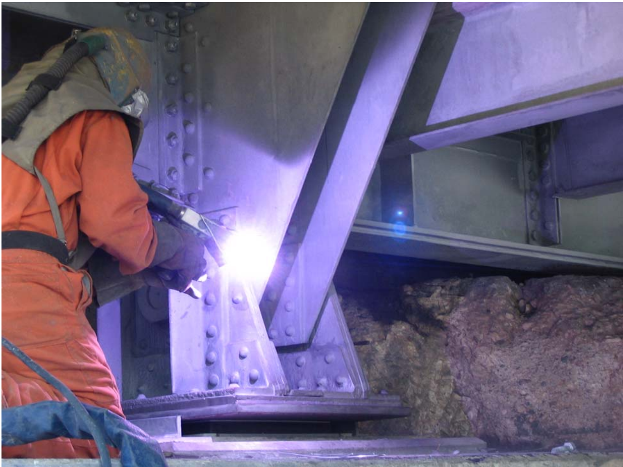
Figure 9. Zinc metallizing process
