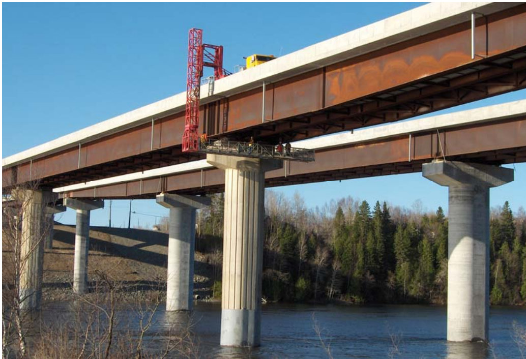
Figure 4 – Biennial structure inspection with specialized equipment
