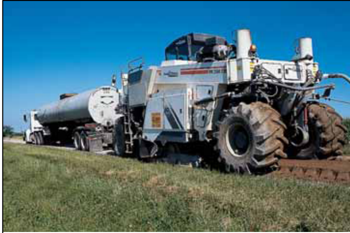
Figure 4.2-2 mixing foamed bitumen with fly ash
