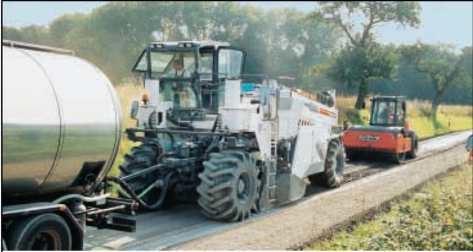
Figure 2.4-2 foamed asphalt being rolled
