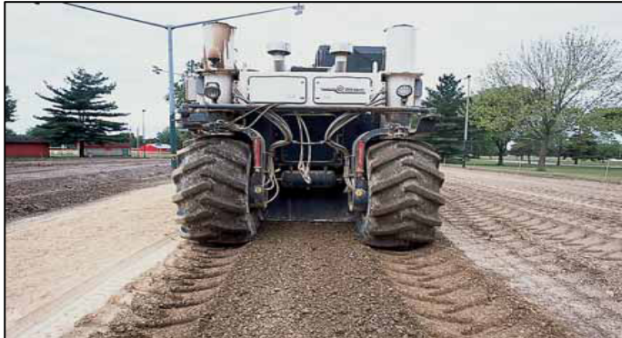
Figure 4.1-2 fly ash mixing process
