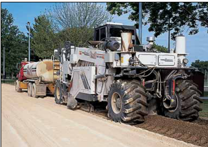
Figure 4.1-1 blending in fly ash with subgrade
