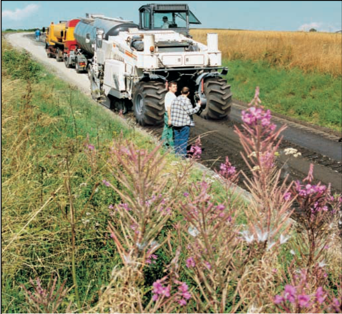
Figure 2.4-1 foamed bitumen stabilization
