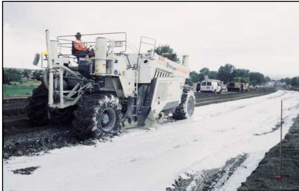
Figure 2.2-1 lime slurry stabilization
