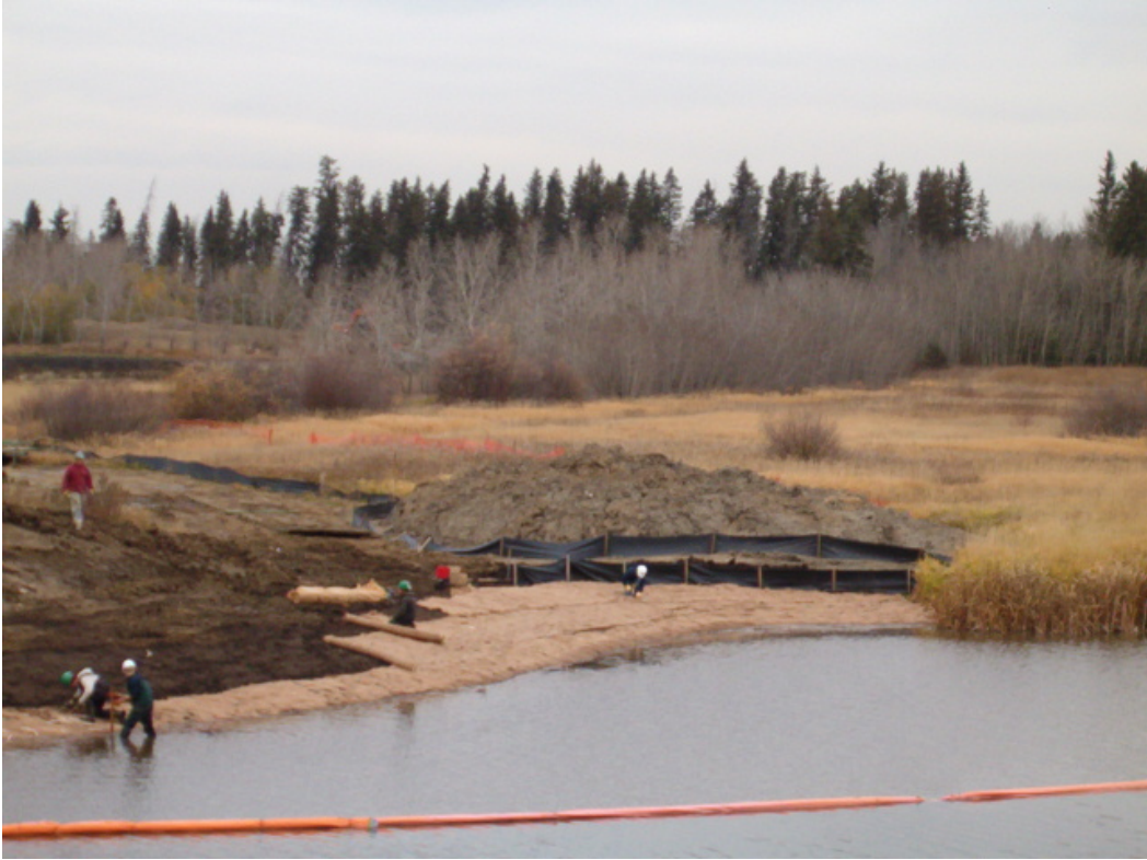
Figure 9: Installation of Coconut Matting Adjacent to Bridge
