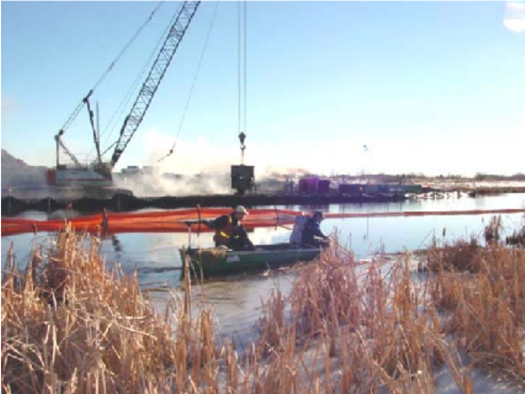
Figure 7: Fish Salvage in North Bank Isolation Area
