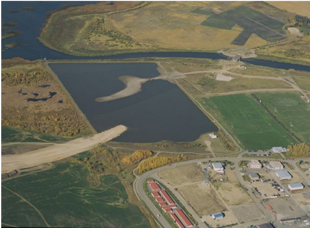
Figure 2: Construction of Sturgeon River Bridge and Causeway over Riel Pond
