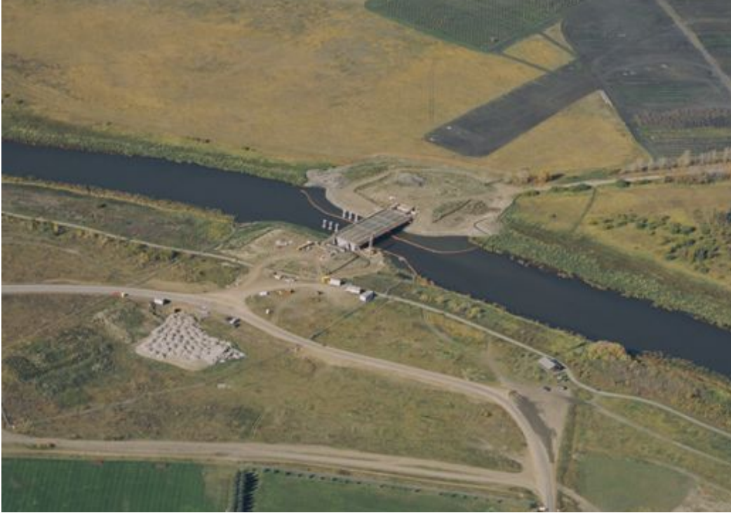
Figure 3: Construction of Sturgeon River Bridge
