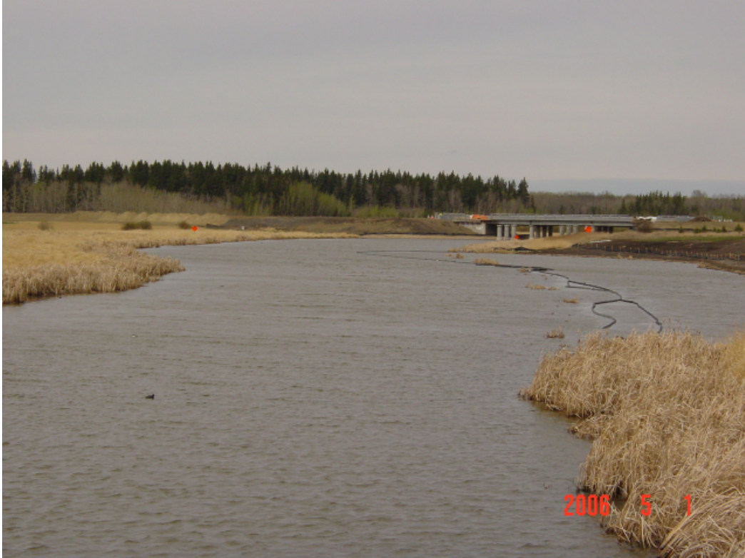
Figure 4: Downstream view of Fish Habitat Compensation Area, Silt Fence in Foreground at 1:5 Year Flood Elevation and Silt Curtain in River (silt curtain approximates former shoreline)
