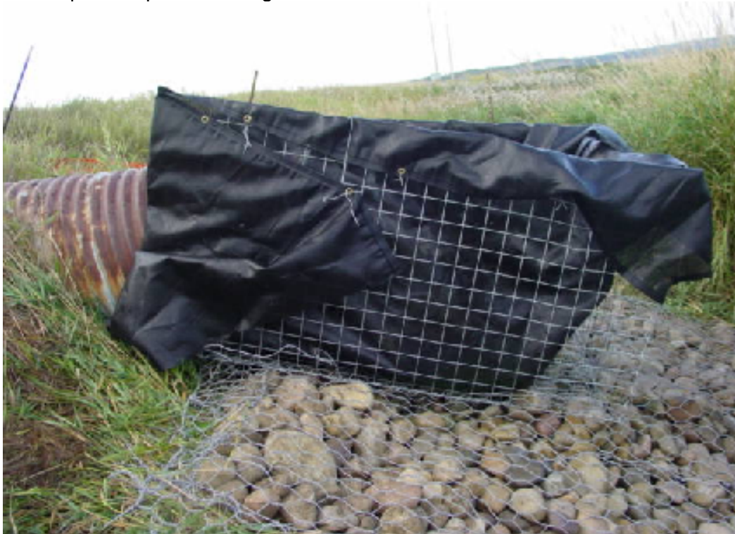
Figure 8: Geotextile-Lined Gabion Basket Filtration Device at Outlet of Riel Pond to Sturgeon River
