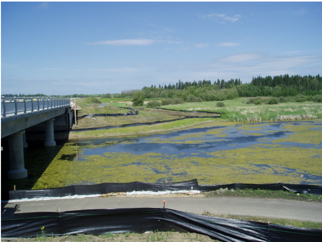
Figure10: Re-vegetated Banks adjacent to Bridge
