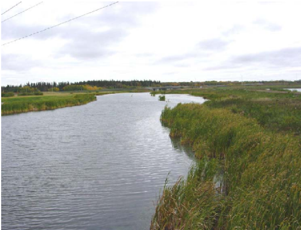
Figure 5: Completed Fish Habitat Compensation Area, Two Growing Seasons Post-Construction
