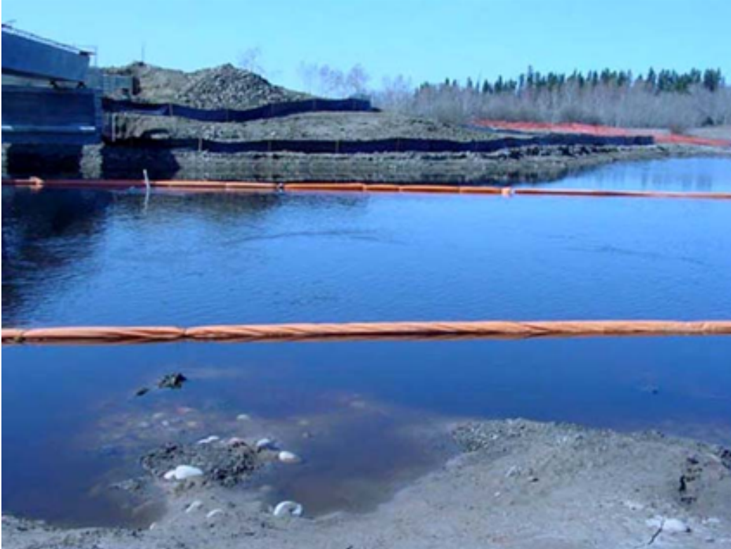
Figure 6: Silt Curtain Installed at Bridge Site
