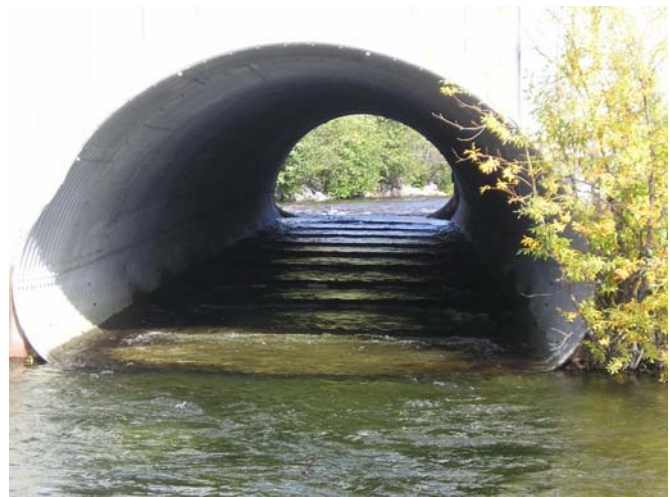
Figure 8. Culvert on left received the baffles; note ice in culverts. The picture on the right shows the baffles in place. Photos T. Omtzigt (YG HPW)
