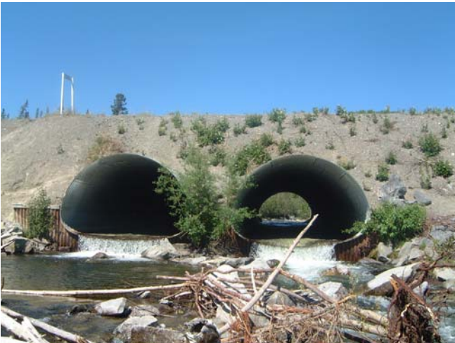
Figure 1. Culverts prior to restoration works. Photo D. Stillwell (YG HPW).
