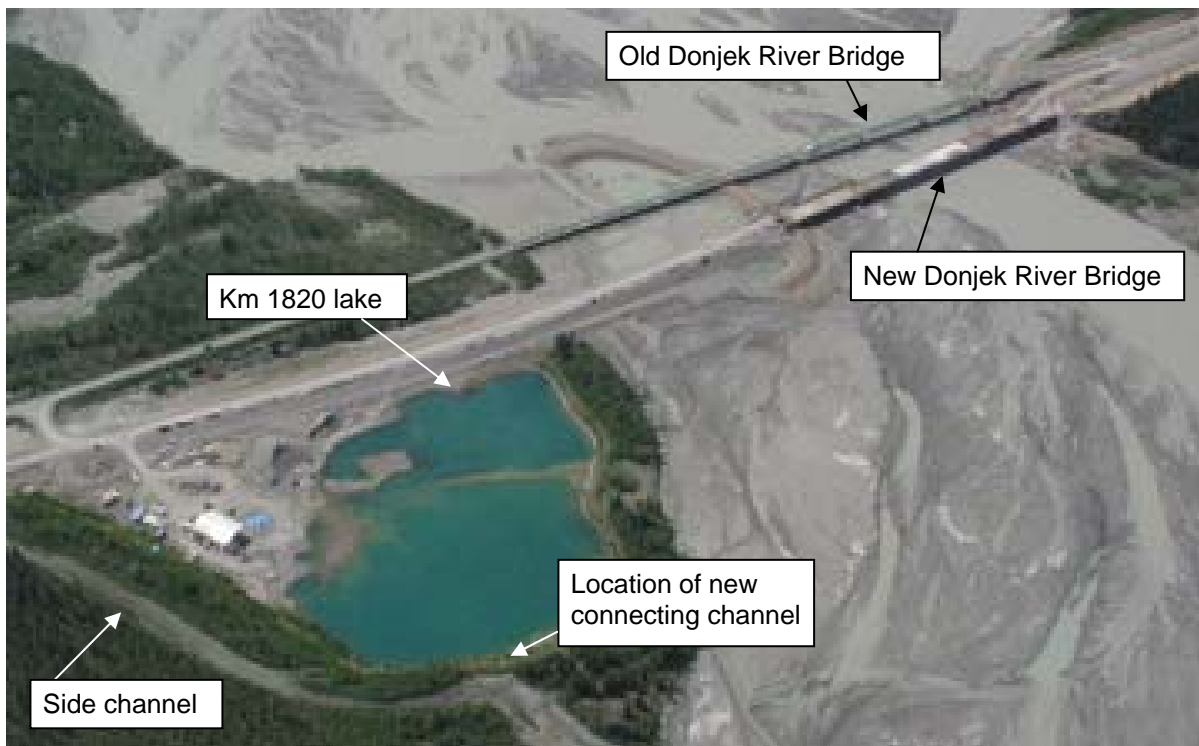
Figure 12: Km 1820 Aerial overview of site and location of new connecting channel. Note color of water in the lake and in the river. (Photo: Google Earth).
