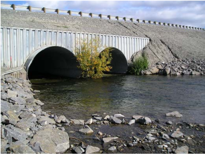
Figure 6. Culverts post construction. Photo T. Omtzigt (YG HPW)
