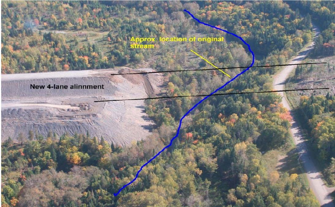
Stream condition after construction – natural vegetation along stream channel and slopes removed along with installation of a permanent stream diversion.
