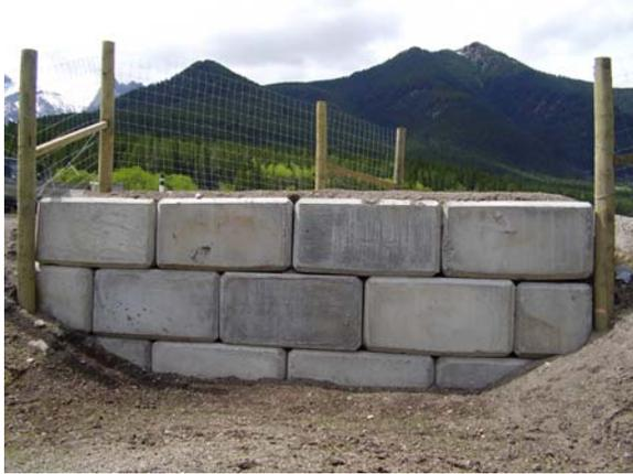
**Figure 9.** Example of a one-way earthen escape ramp planned for use in the wildlife exclusion fencing system – Deadman Flats, Alberta.
