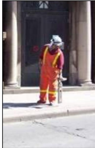
**Figure 3 - Field Technician using Cable Locate Equipment**
