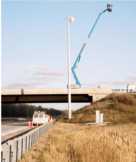
Figure 6 - Installation of Wireless Equipment at Camera Site in Sarnia
