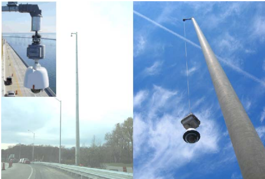
Figure 4 - Dome CCTV Cameras with Lowering Device Installed on Hwy 402
