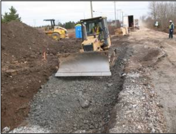
Figure 14a & 14b – Placement and Compaction of Foundation Improvement Material – Stage Two
