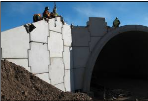
Figure 9a – Permanent MSE Wall Photo
