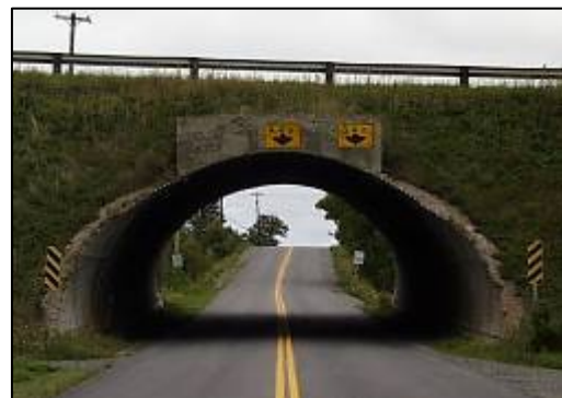
Figure 1b – NSTPW Existing Structure
