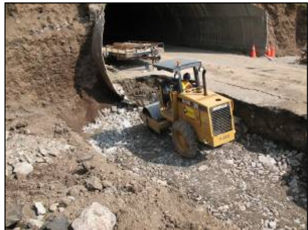
Figure 12b – Compacted Engineered Fill South End
