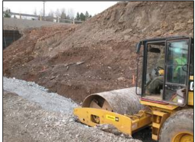
Figure 14a & 14b – Placement and Compaction of Foundation Improvement Material – Stage Two
