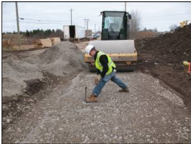
Figure 15a & 15b – Compaction Testing Foundation Improvement – Stage Two
