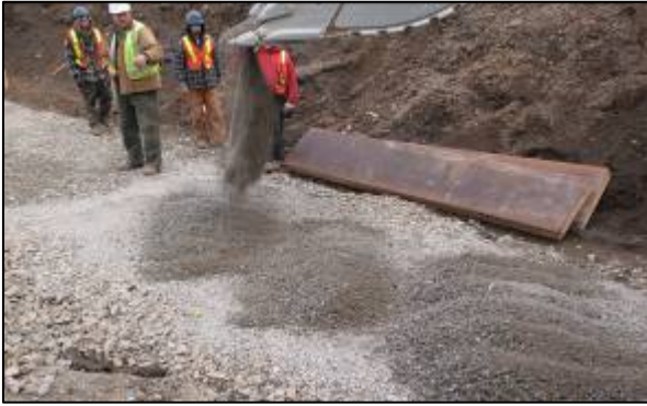
Figure 16a – 19 mm minus Granular Placement
