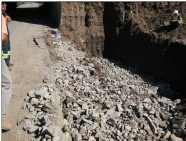
Figure 12a – Placement of Engineered Fill South End
