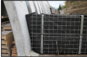
Figure 8a – Temporary MSE Wall
