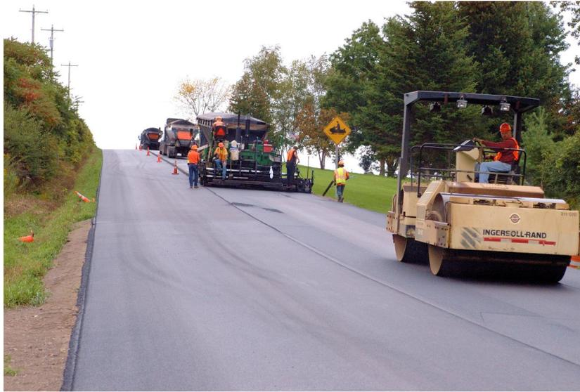
Photo 1 – Warm mix asphalt paving operation
