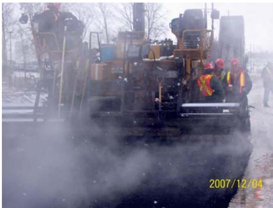
**Figure 10 – Paving Oxford Road 4 in Dec 2008**
