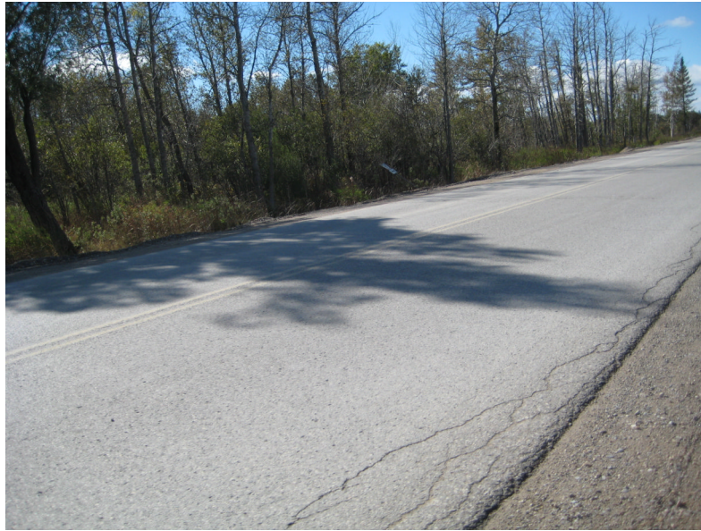
Photograph 3 The pavement on the east part of County Road 11 was relatively intact with only low severity cracking.
