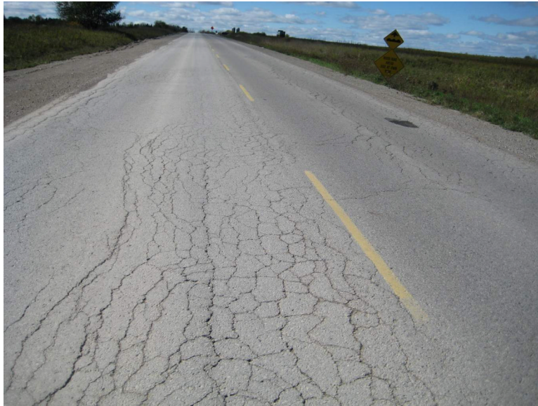
Photograph 1 High severity alligator cracking area on west part of the existing pavement on County Road 11.
