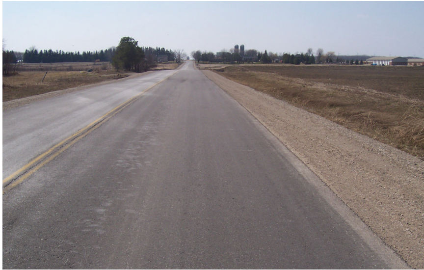
Photograph 11 Pavement condition in April 2008.
