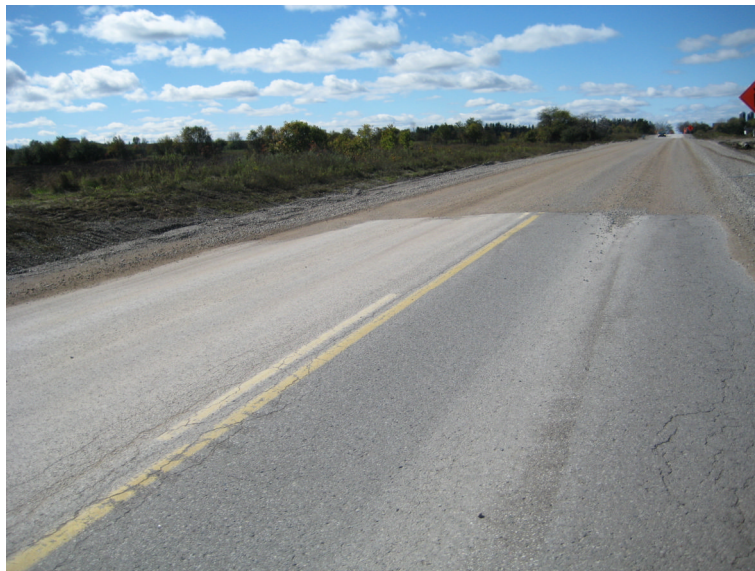
Photograph 2 The pavement was repaired with new granular material before foamed asphalt stabilization in areas exhibiting the most severe alligator cracking.
