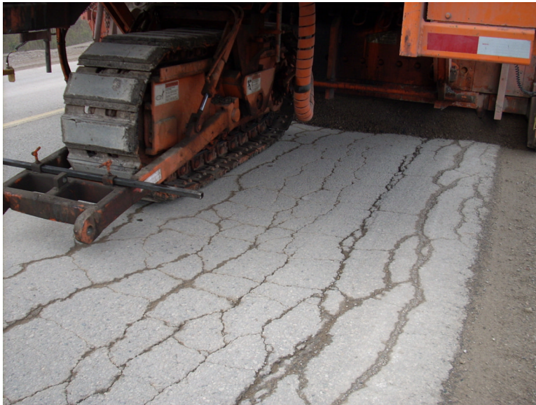
Photograph 5 Areas exhibiting severe alligator cracking being foamed asphalt stabilized.
