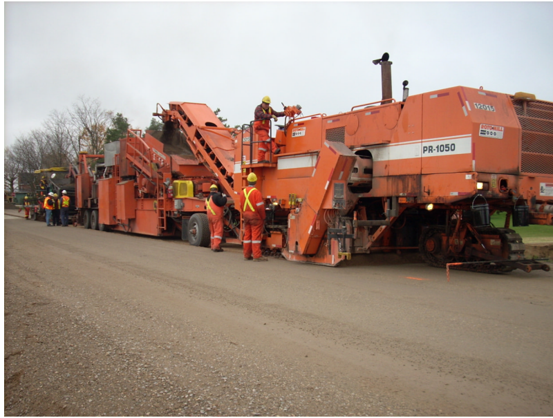
Photograph 4 The recycling train working on County Road 11.
