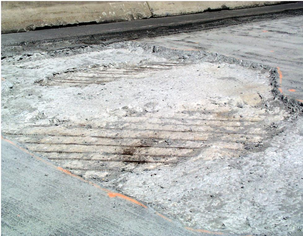
**Figure 11 Localized corrosion of rebar over circular voids of PT deck**
