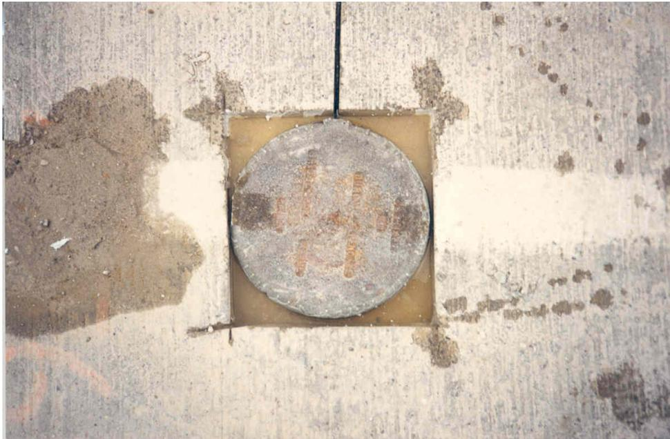
**Figure 3 Pancake anode recessed into concrete deck**
