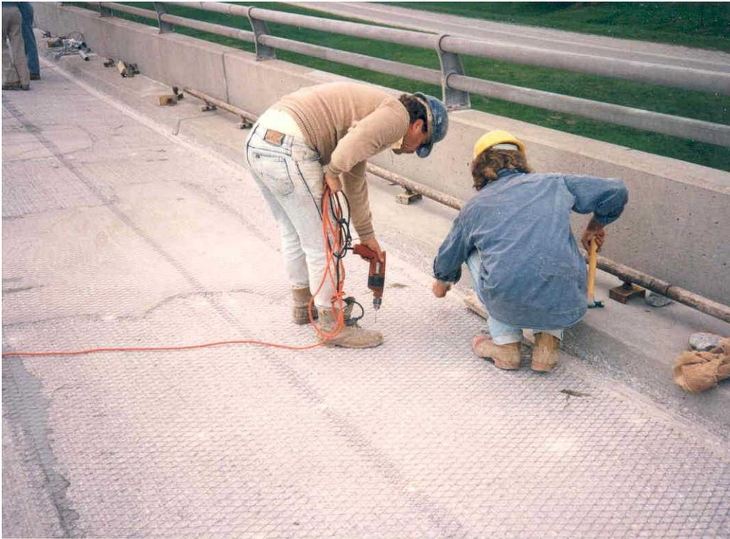
**Figure 13 Titanium Mesh Anode Cathodic Protection System**
