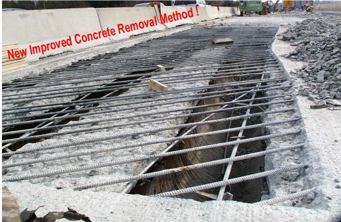
Figure 16 Excessive concrete removal of a post-tensioned deck with circular voids
