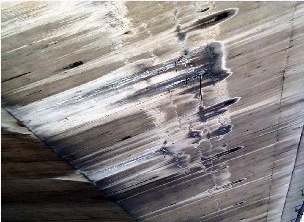
**Figure 6 Soffit of Post-Tensioned Deck with leaching cracks**
