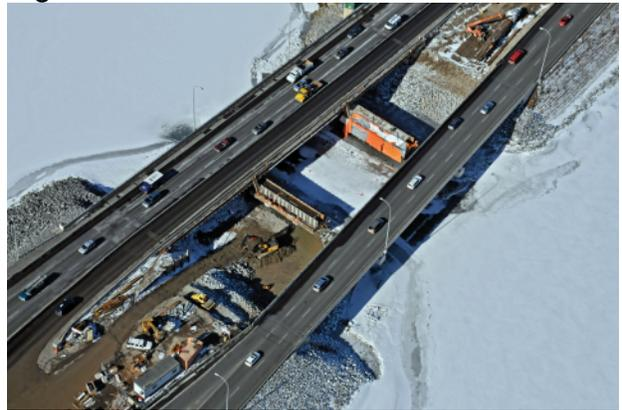
Figure 29 – WB Bridge False Deck
