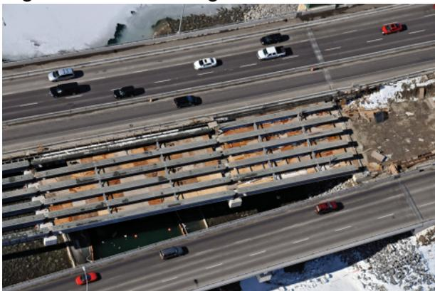
Figure 30 – WB Bridge Deck Formed
