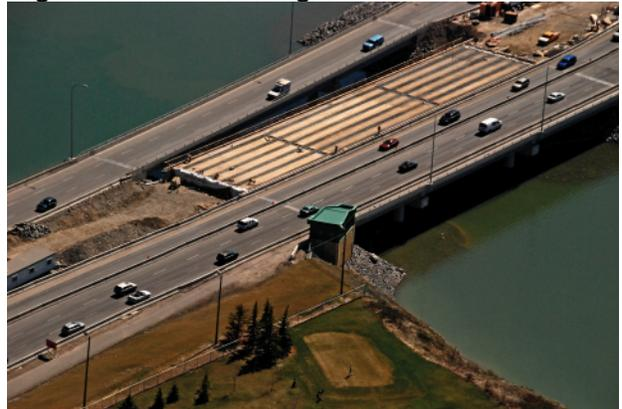
Figure 31 – WB Bridge Deck Pour
