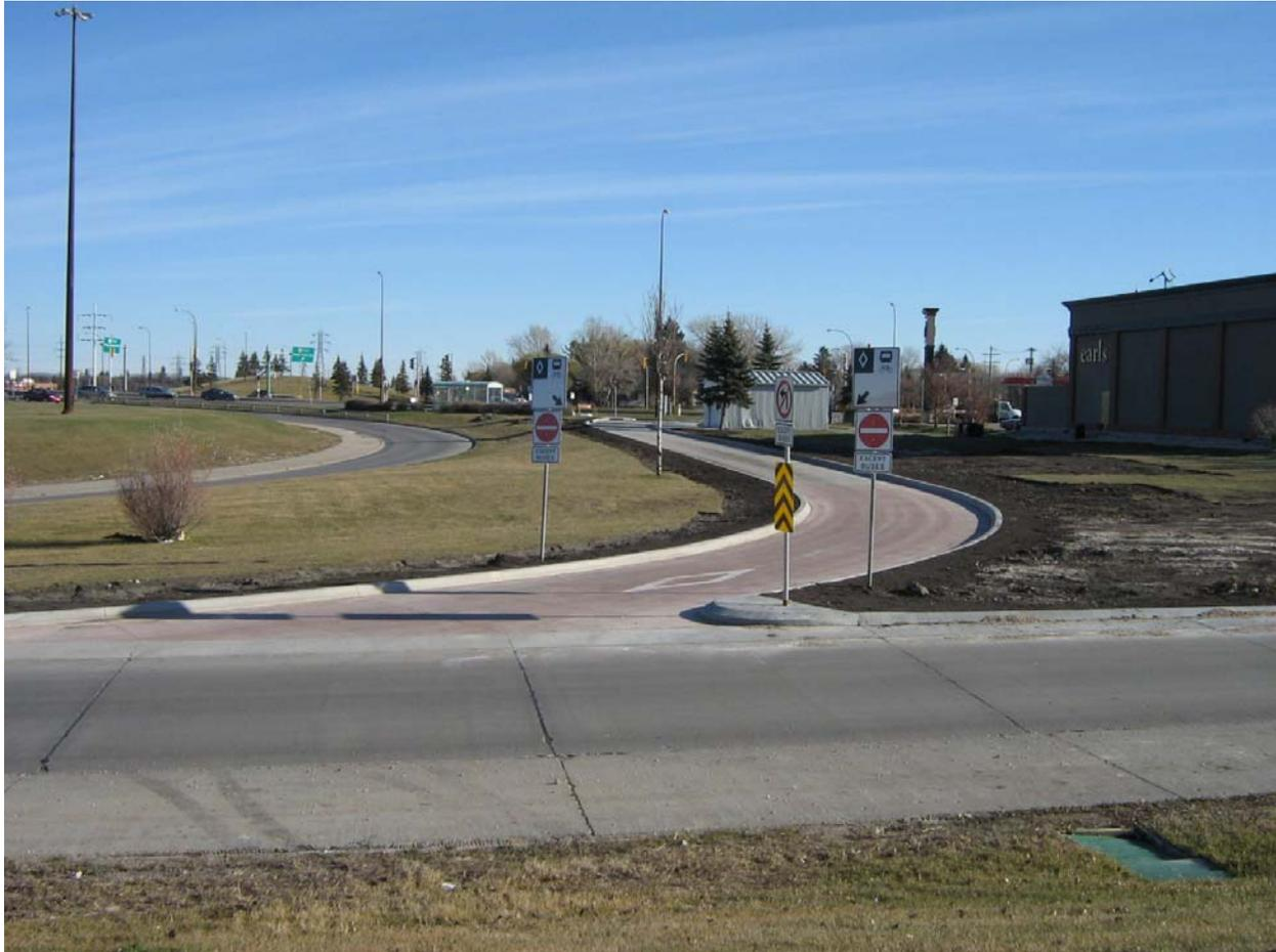
***Pembina Highway Corridor*** - As with many of the other queue jumps and transit priority signals installed, the northbound Pembina at Jubilee measure occurs at a constriction point. Here, the northbound lanes constrict from three to two, and allow buses to remain in the curb lane and bypass the regular traffic queue with a transit priority signal.
